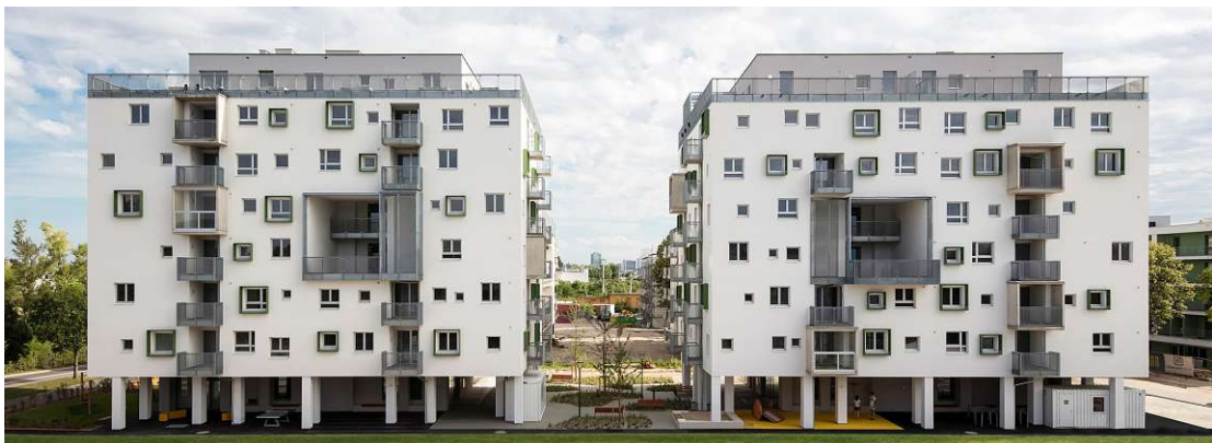
Figure 5. North facade (Hawelka 2020)
