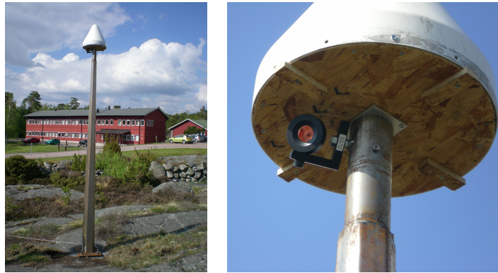
(a) Mast construction (b) Prism mounting at the top of the mast
