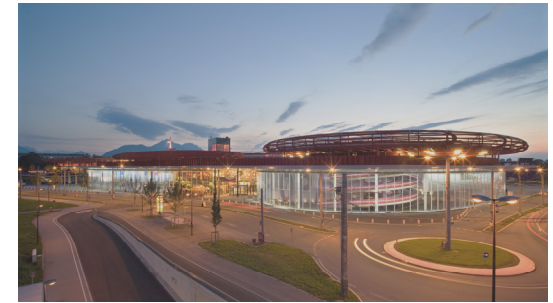
Abb. 3: Europark, Fassade, Arch. Massimiliano Fuksas
