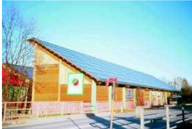
Figure 15: picture of district heating system Eibiswald (energytech, 1998)
