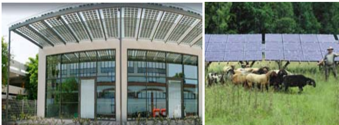
Figure 9: Multiple shift usage – shading by photovoltaic panels and sheep paddock with photovoltaic installation
