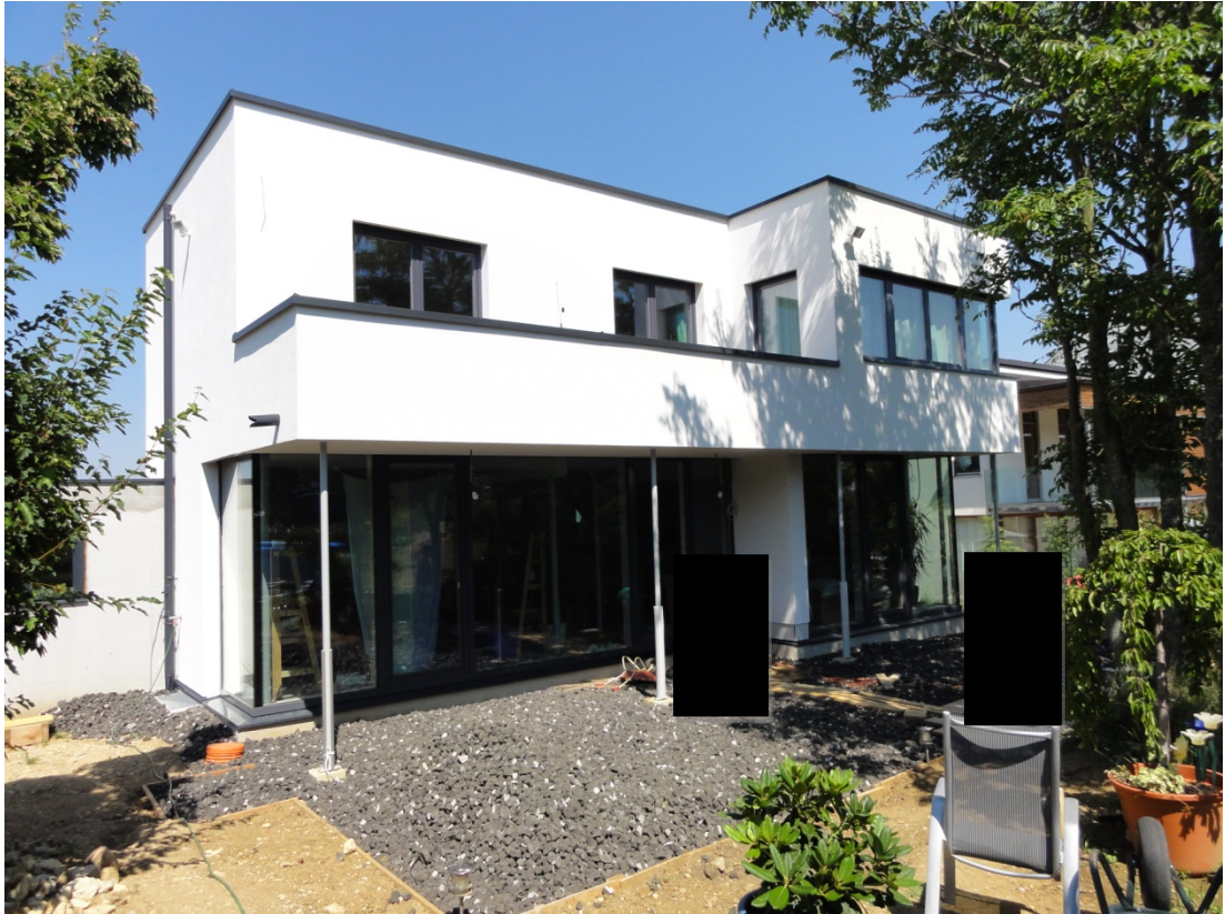
Figure 16: garden-view to the building (Baden) – own photograph
