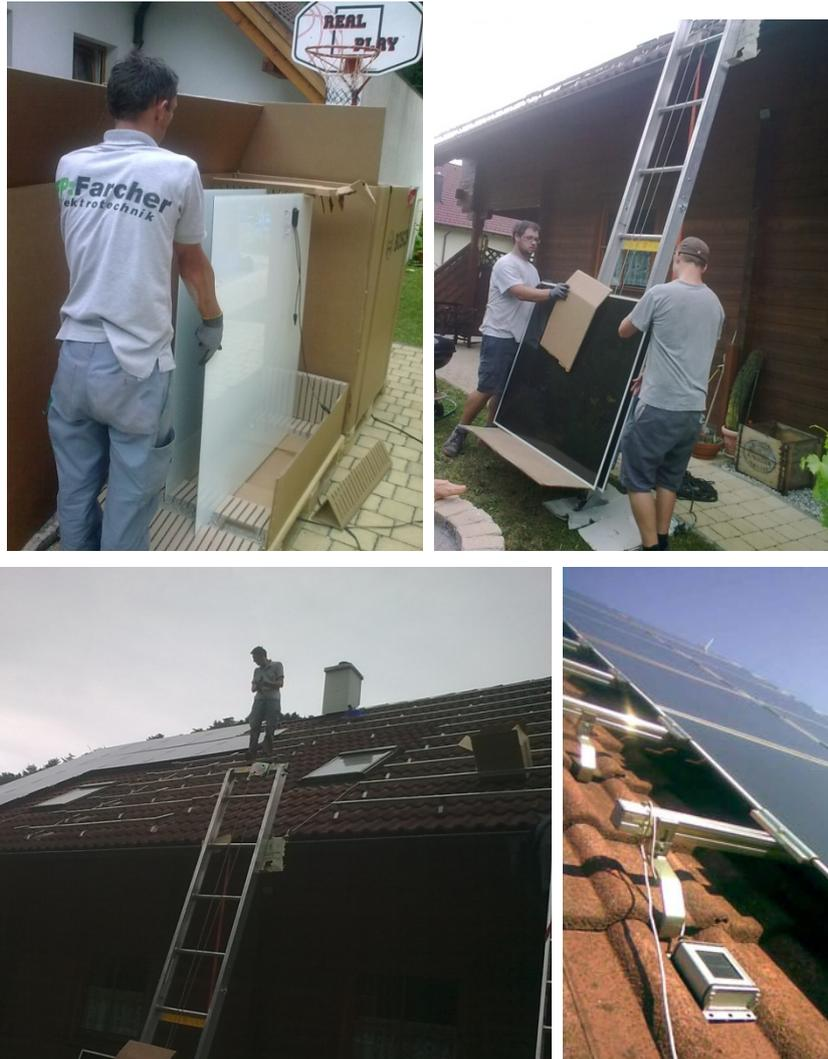
Figure 10: It was important to make the initial measurement right after the installation. This way we could measure the highest productivity of the panels before the light induced degradation had affected the cells. The pictures show the installation of Bosch  $\mu$ -Si plus 115 in Gutenstein and the irradiation measurement.
