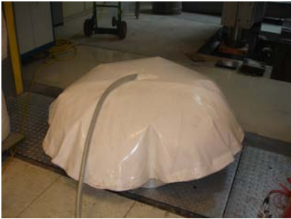
Figure 70: Inflated pneumatic formwork
