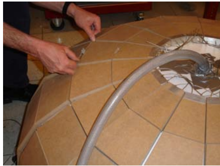
Figure 73: Manual adjustment of the ring cables
