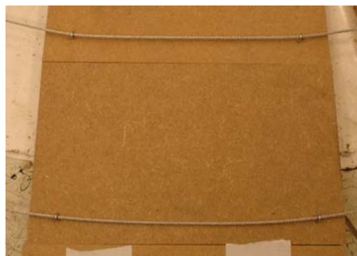
Figure 79: Placement of the ring cables
