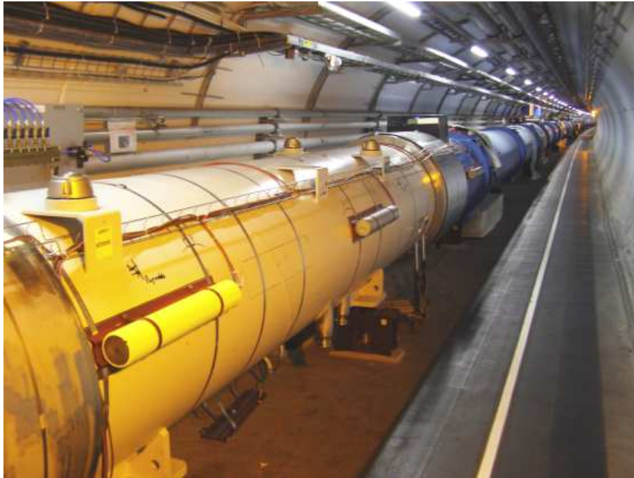
Figure 1.2: Installation of the LHC BLM system detectors outside a quadrupole magnet.
