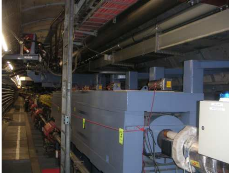
Figure 6.3: Detector installation on the HERA proton beam dump.
