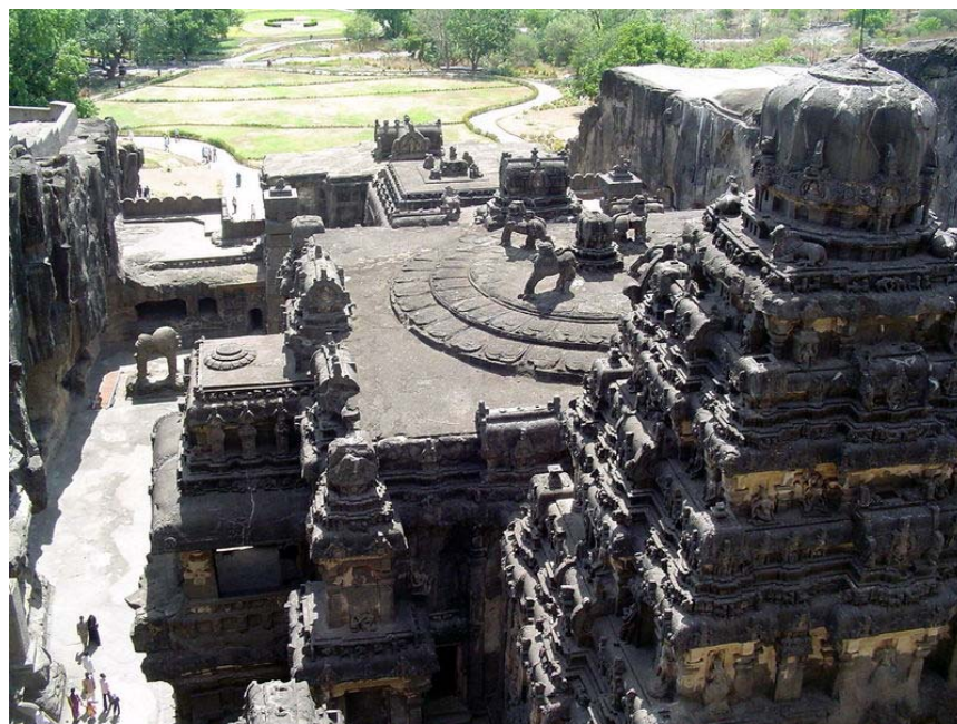
Picture 98, 99 & 100, Kailash Temple - the largest monolithic structure in the world
