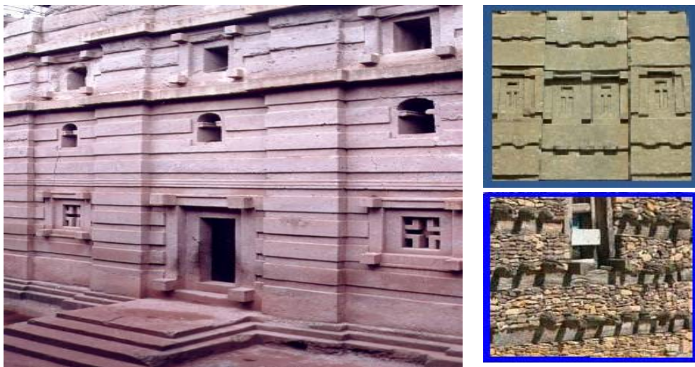
Picture 32, a view of the façade of Bete Amanuel and a section of the façade of an Axumite Stele and Debre Damo church showing the typical Axumite stone-wood architecture
