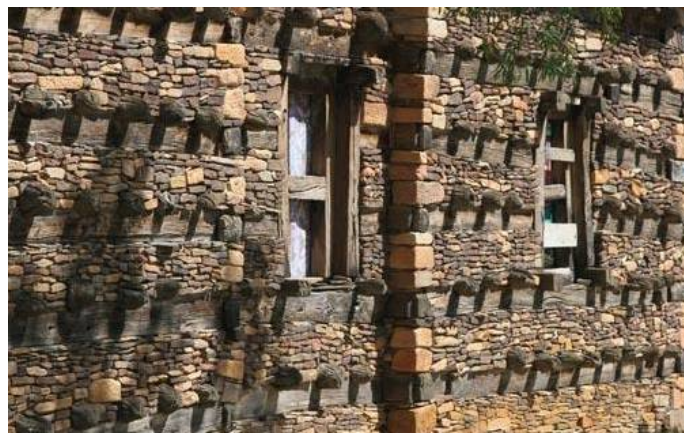
Picture 59,60 & 61 Front, façade & interior of Debre Damo Church the oldest existing Axumite church (Altered Tin roof) showing the combination of wood and stone in Axumite architecture
