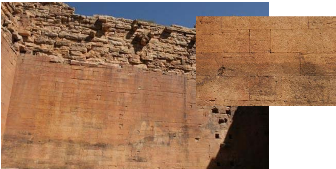
Picture 54, Details of construction with a fine surface finishing at Yeha Temple
