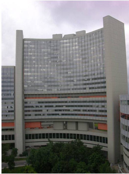
Figure 2.1-4 General view of north façade of tower D (building VC)
