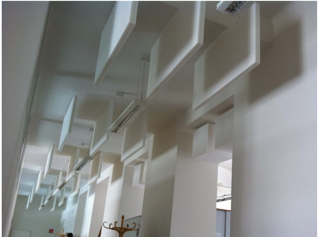
Figure 32 OP after retrofit
