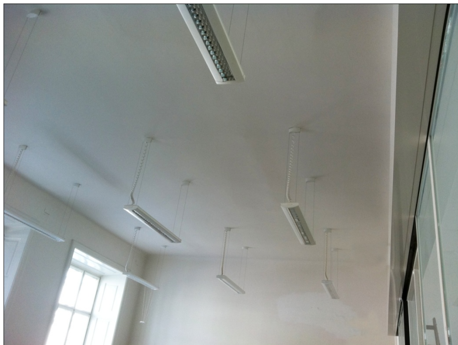
Figure 11 Existing conditions in SR
