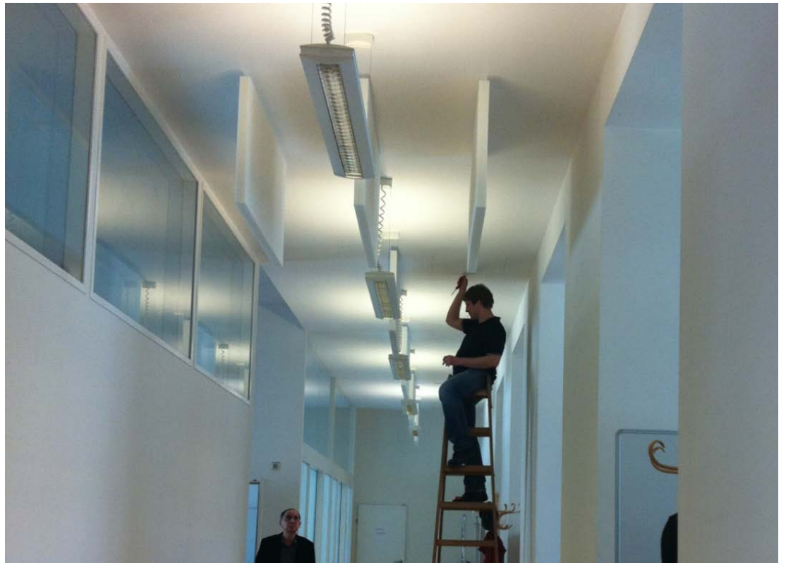
Figure 30 Mounting process of absorber elements
