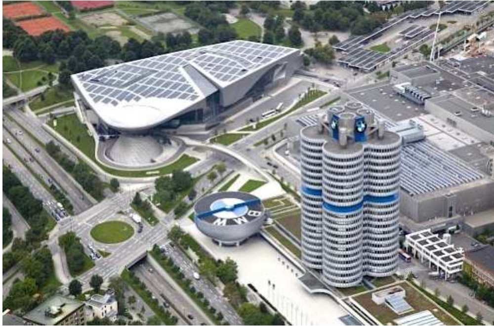
Fig.44 BMW Welt Munich PV power plant (Source: BMW GROUP)
