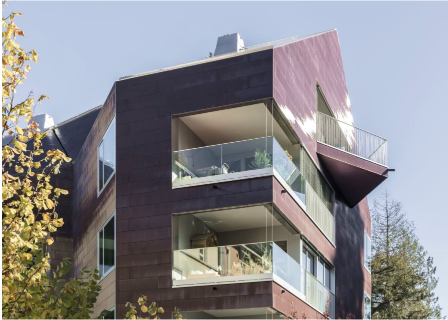
Fig.47 The most innovative Residential BIPV project. Zurich, Switzerland Image Courtesy © Beat Buhler
