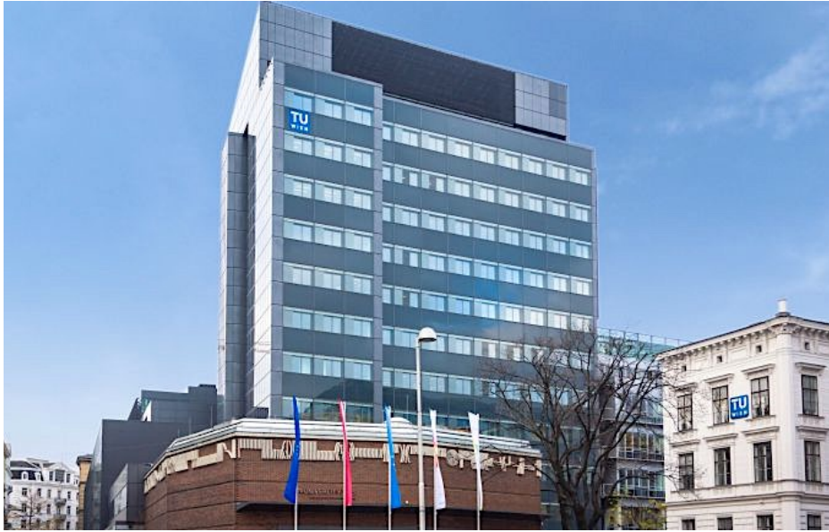
Fig.48 Energy plus office tower (TU Wien) in Vienna Image courtesy © Schöberl & Pöll GmbH
