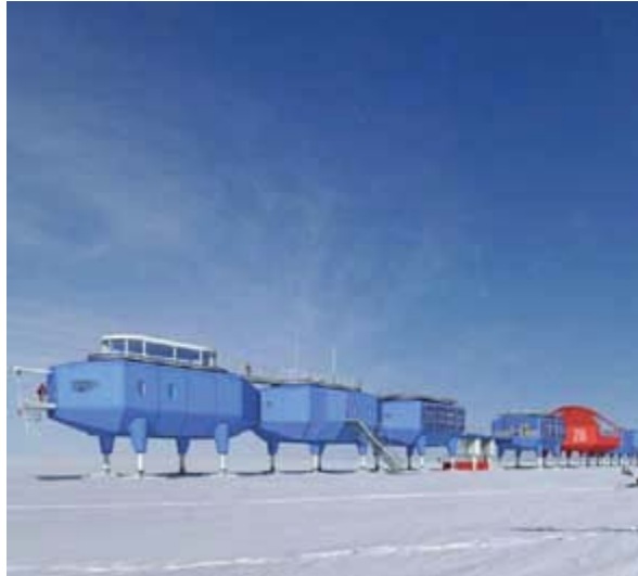
Figure 3-6: Halley IV Antarctic station. Elevating the structure for protection against environmental hazards is also applicable in terrestrial extreme environments. (Credit: Hugh Broughton architects)
