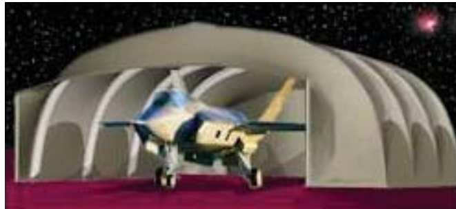
Figure 3-18: An artist's impression of the currently developed inflatable aircraft hangar. The rapid deployment and dismantling of the unit is a critical design driver, in regard to the military use. (Source: US Air Force Materials and Manufacturing Directorate)
