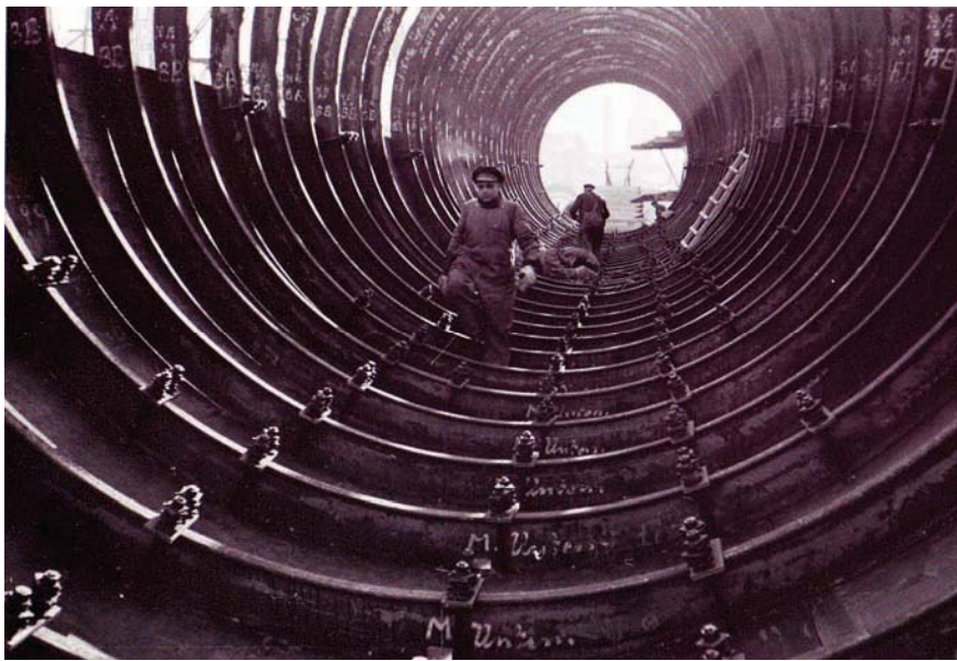
Figure 3-40: A submarine under construction in Germania Werft, Kiel. The main envelope for the spatial arrangement of a submarine vessel is dictated by the hull structure (Credit: Kaplan)
