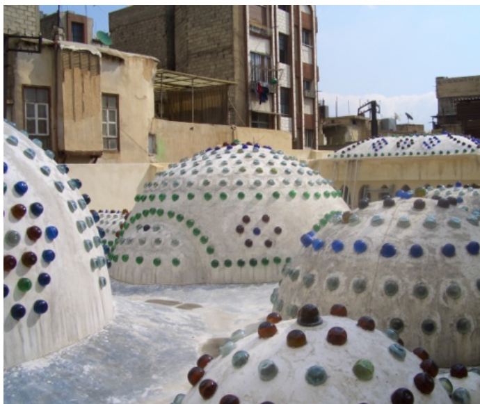
Figure 8 Typical openings in domes of hammam, outside view (Hammam Fairouzi)
