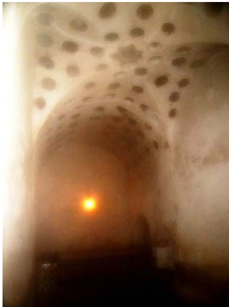
Figure 236 Deterioration of daylight and fresh air supply to the interior spaces of a hammam in Fez (Morocco) due to the blockage of roof apertures
