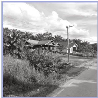
DOUBLE ROOF VERANDAH
