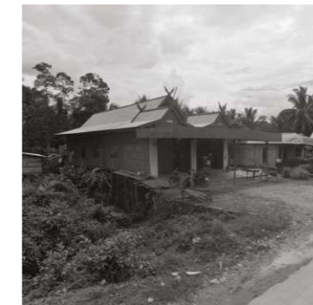
2 Bugis Roof finishing
