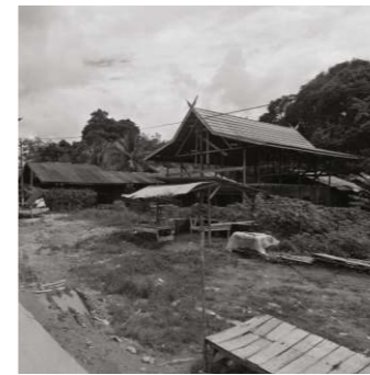
1 Bugis roof finishing
