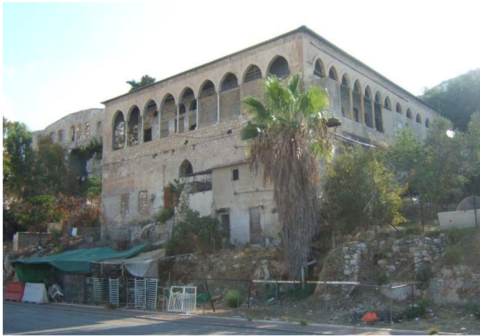
Figure 2.2.7: The eastern façade of the house at 19 Ma'ale Ha-Shihzur Street (photo taken by the author, 2011)
