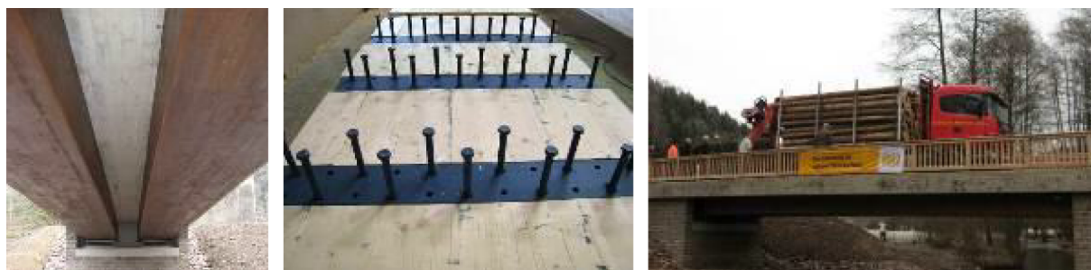
Abb. 2.4: Birkbergbrücke in Wippra [6]
