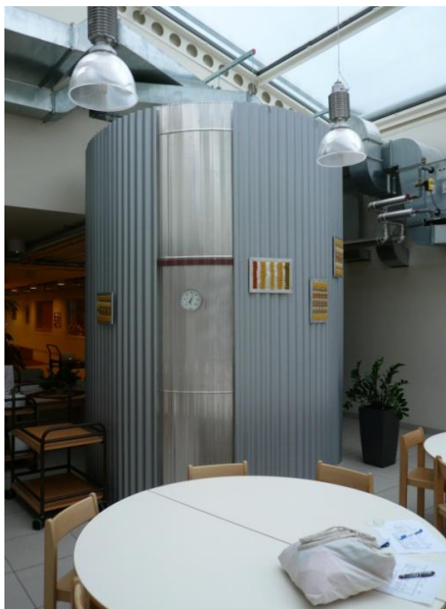
Figure 10: Domestic hot water tank in the atrium of the PHKG.
