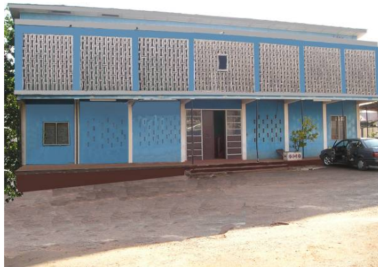
Fig.21: External view of building DCD
