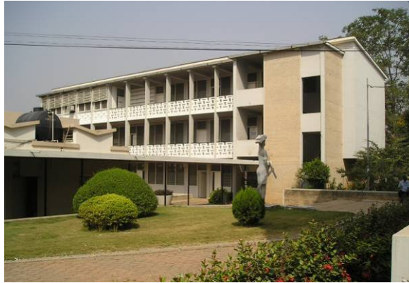
Fig.1: External view of building CAP
