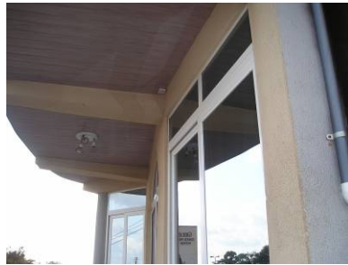
Fig.17: Cantilevered overhang above the entrance
