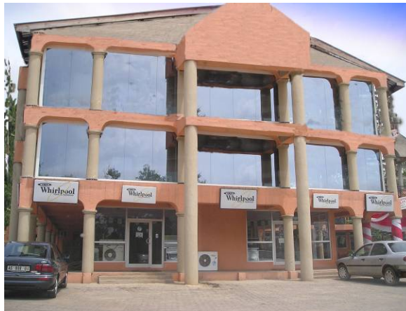
Fig.18: External view of building ROY
