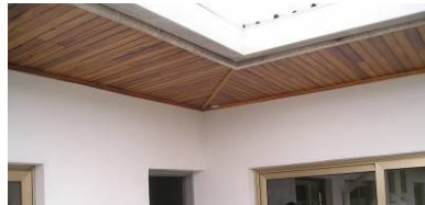
Fig.11: Overhang, partly shading exposed windows
