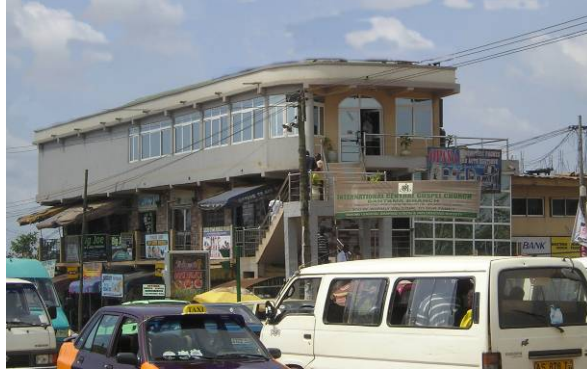
Fig.12: External view of building ANG
