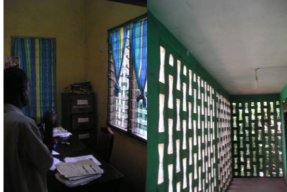
Fig.24: Sample office with the shading veranda
