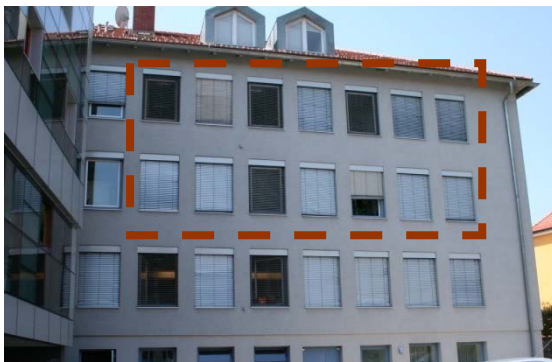
Figure 2-17 General view of observed offices
