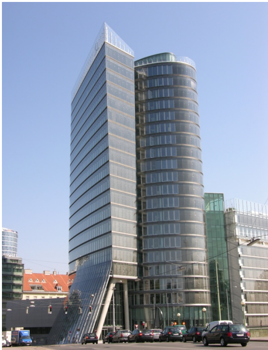
Figure 2-11 General view of UT from South
