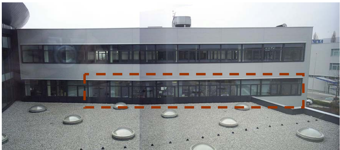
Figure 2-7 Observed area of ET façade, View from East
