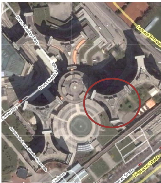
Figure 2-1 Aerial view of VC; tower D
