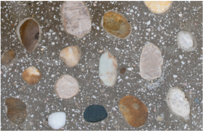
I The outer facade is made out of Riverstone Concrete slabs that are cut to size. Due to the abundance of oak in the region, the interior is covered with oiled oak plywood and oak floor boarding
