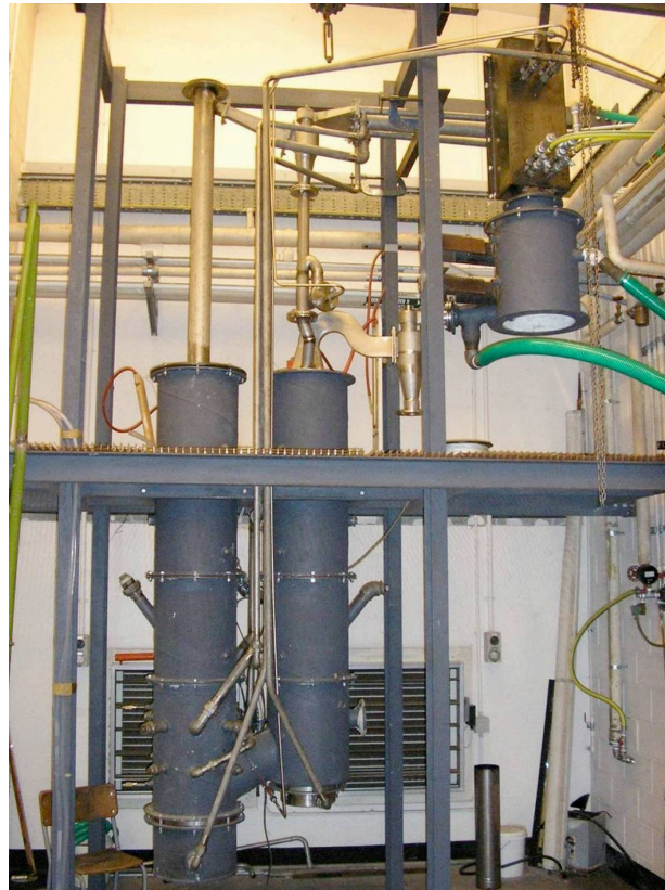
Figure 6.3: Gasifier without insulation [22]
