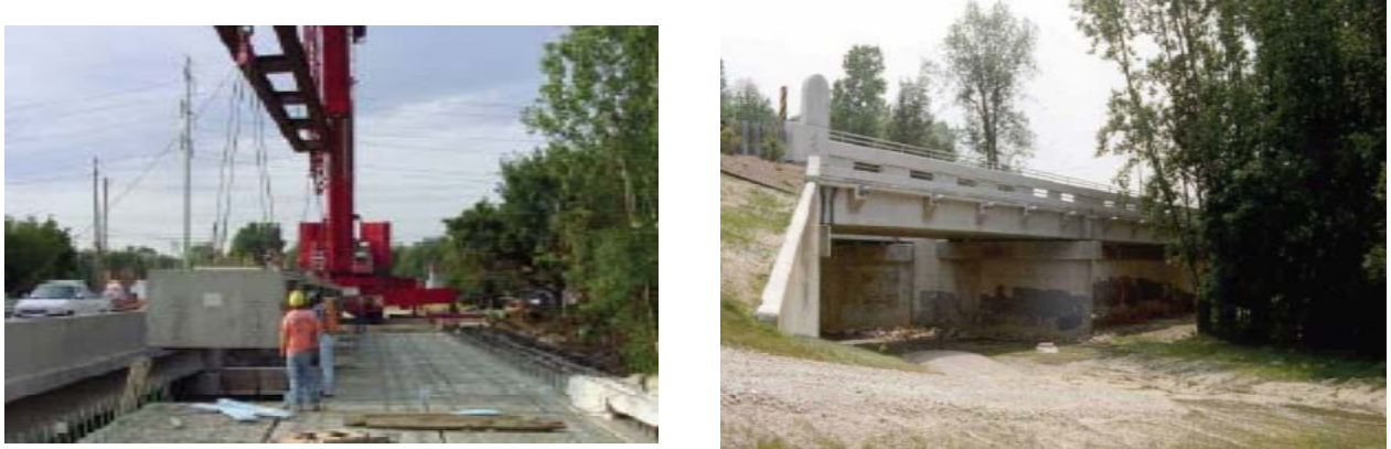
Abb. 9: Bridge Street Bridge [www.ovbb.at]
