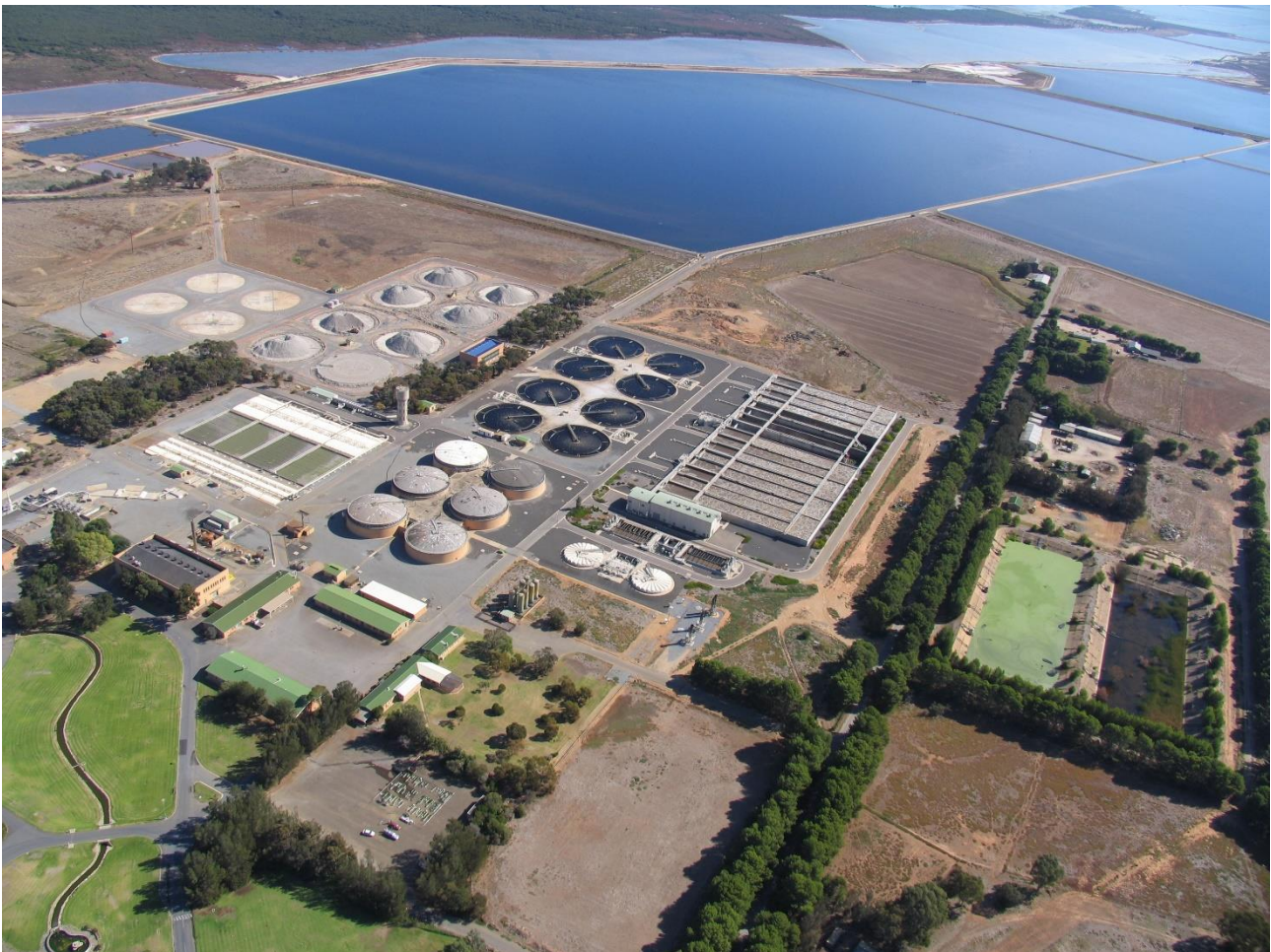
Figure 2: Aerial photograph of Bolivar WWTP not showing the sludge lagoons, hardstand and stockpiling area
