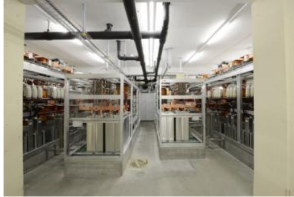
Figure 7-13 Frequency converter of Grimsel 2 143
