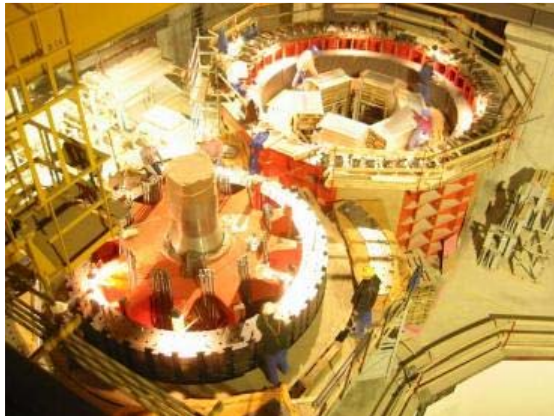
Figure 7-6 Machine units DFIM(left) and SM(right) of Goldisthal 135
