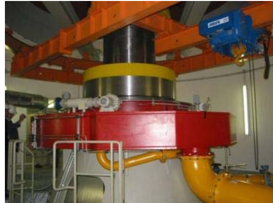
Figure 7-7 Trust bearing of Goldisthal 135
