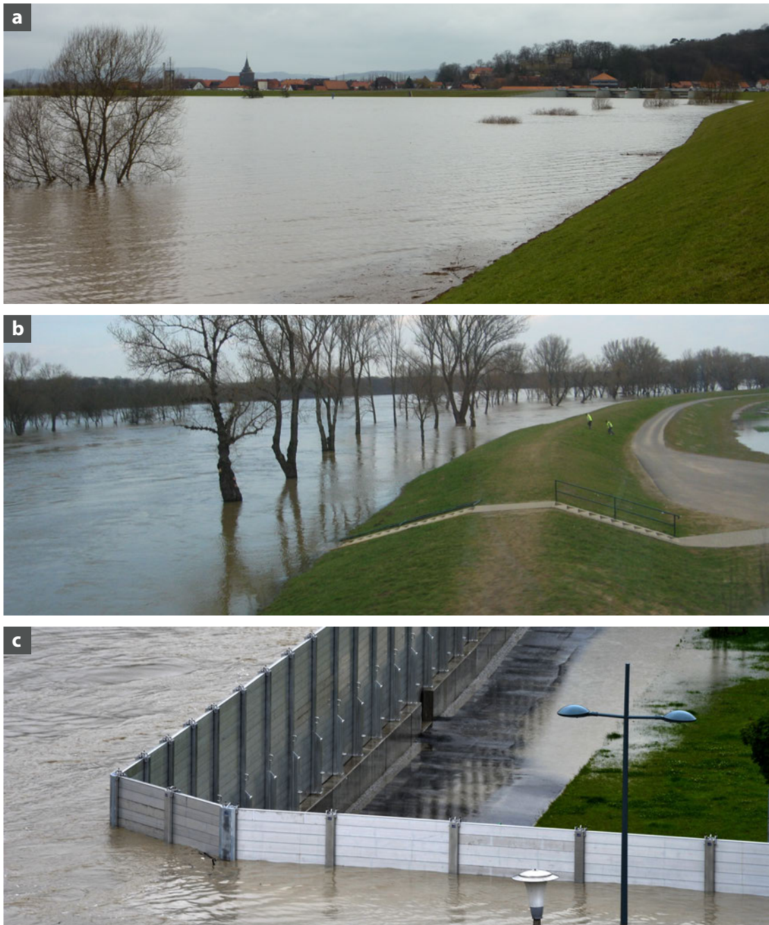
Figure 1.3: Examples of long-term flood protection measures. (a) Retention areas. (b) Dikes. (c) Floodwalls.
