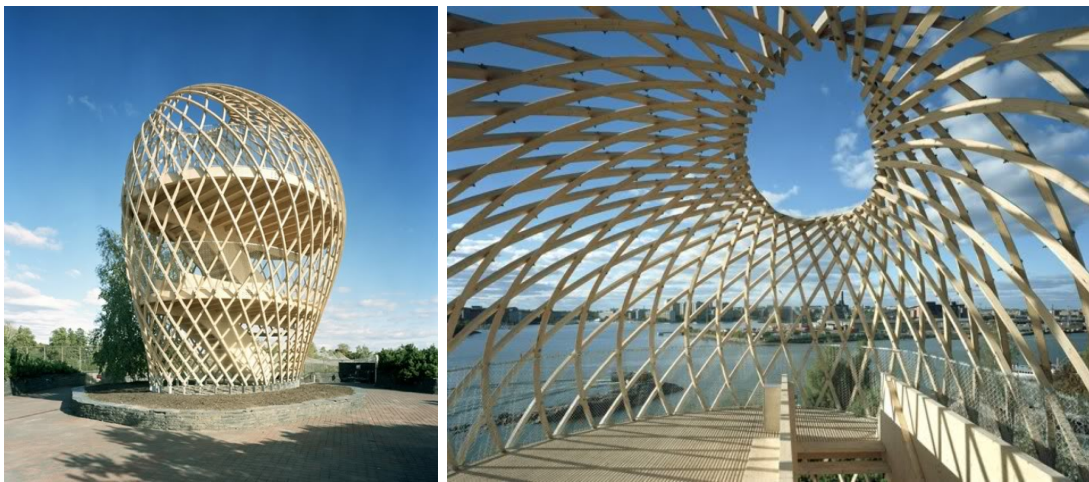
Figure 3.4: The Korkeasaari Lookout Tower in Helsinki, Finland, with the outer shell built from laminated timber beams. Photos by Jussi Tiainen.
