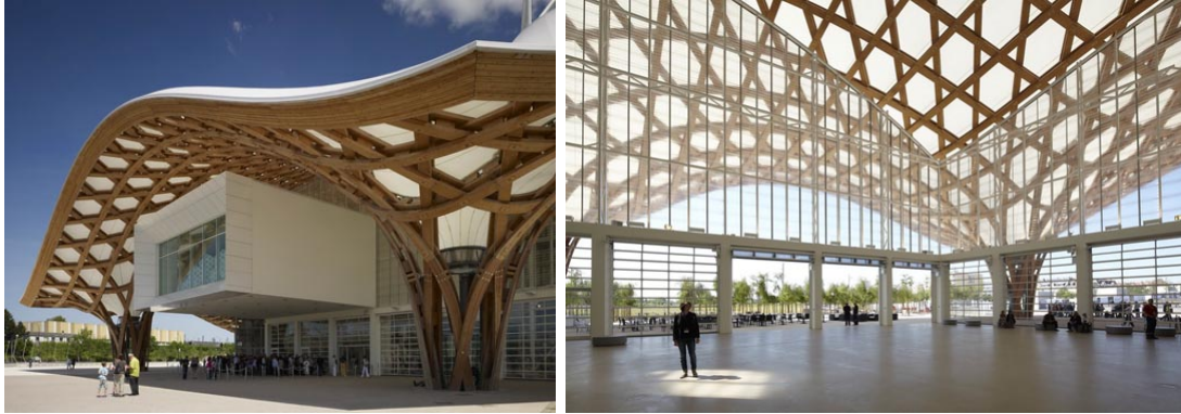
Figure 1.4: Centre Pompidou-Metz, France, designed by Shigeru Ban. The roof contains an interwoven curve structure made from glued laminated timber. Photos by Didier Boy de la Tour.
