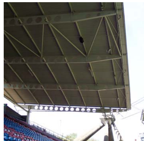
Fig. A-15: The triangular shaped truss, the rafter spanning from the trusses to the rear of the stands, and the corner support.
