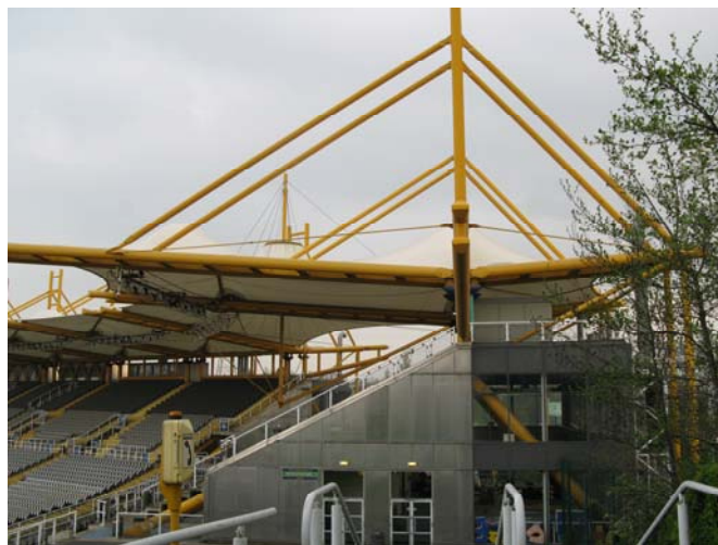
Fig. A-11: Cantilever roof structure supported at the rear of the stand
