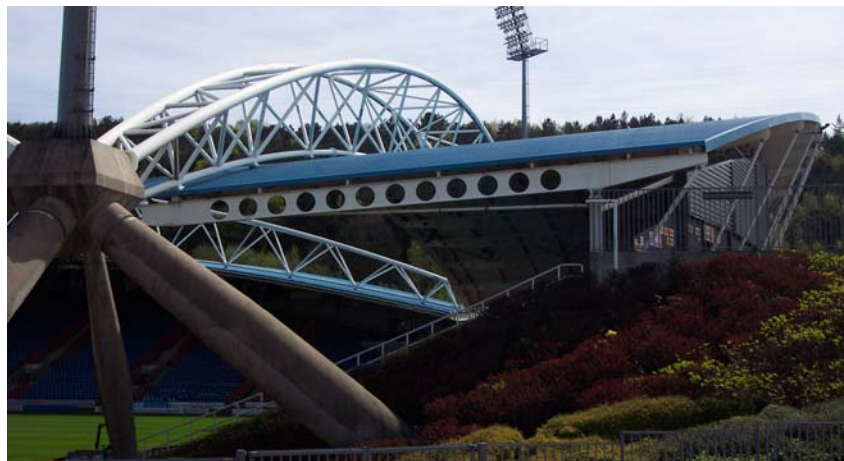
Fig. A-15: The triangular shaped truss, the rafter spanning from the trusses to the rear of the stands, and the corner support.
