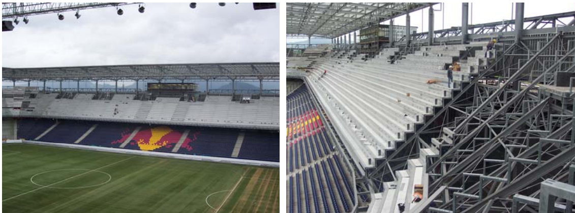
Fig. 3.6: left: Permanent lower tier and temporary upper tier with roof lifted into a higher position; right: Temporary upper tier made of steel with aluminium seating rows
