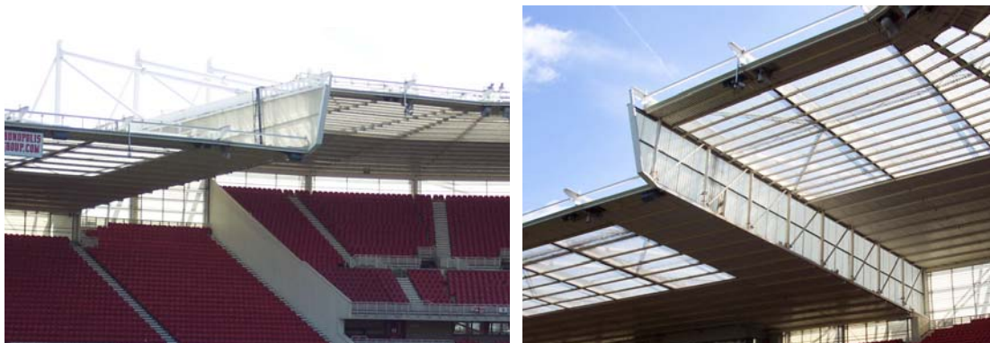
Fig. A-47: Change of level in the roof between the South and West Stand.
