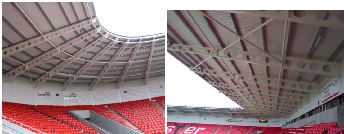
Fig. A-24: Roof structure from inside
