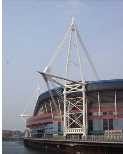
Fig. A-31: Corner mast of roof structure
