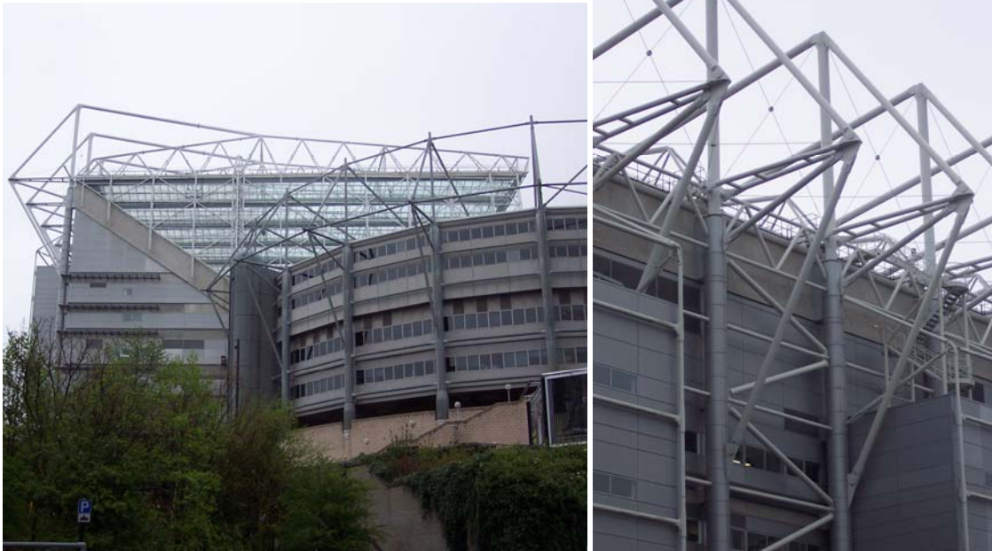
Fig. A-49: Roof structure of the Milburn Stand
