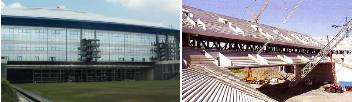
Fig. 3.21: Veltins Arena : left: Gate for movable pitch; right: Under construction [42], [43]
