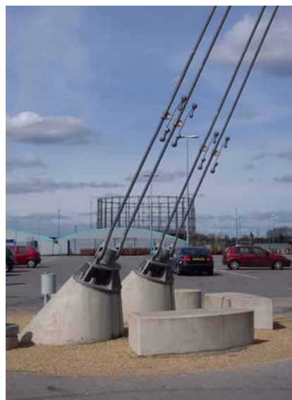
Fig. A-7: foundation of one of the backstay cables
