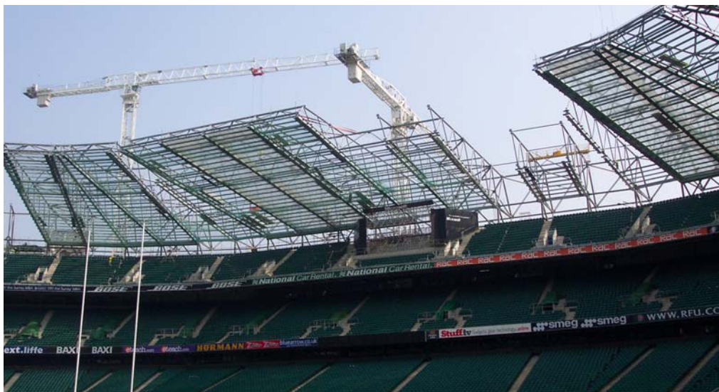
Fig. A-51: Roof of the south stand under construction.
