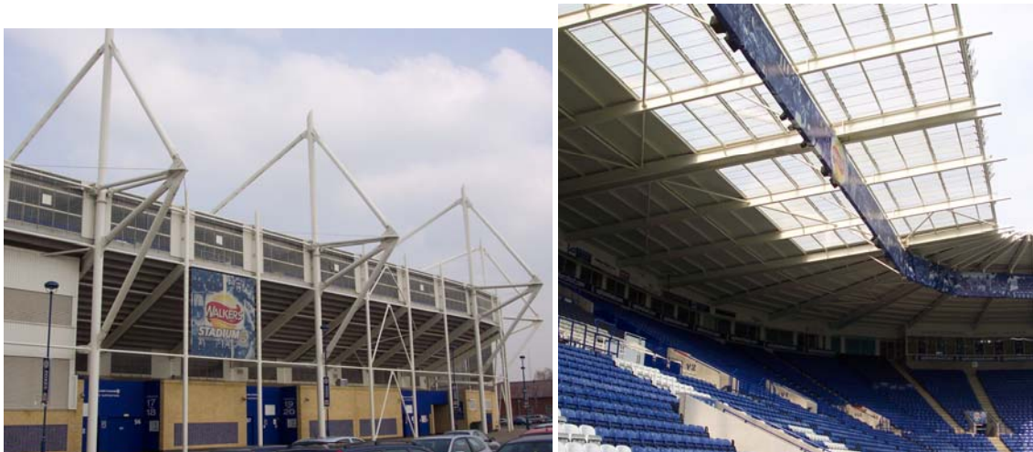
Fig. A-53: Roof structure from outside (left) and inside (right)
