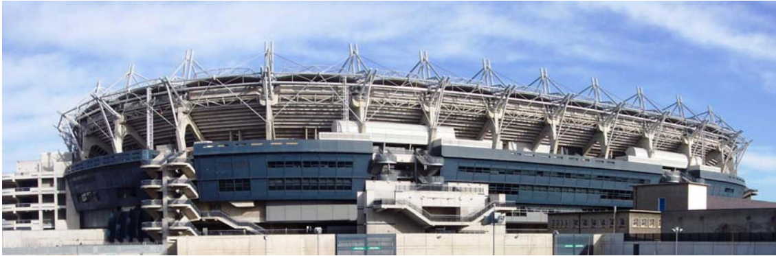
Fig. A-8: Croke Park from the outside, showing the supports of the cantilever roof structure
