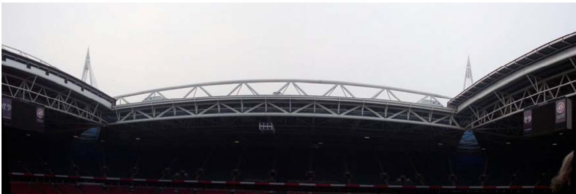
Fig. A-32: Main truss (the support for the retractable roof elements) with the tops of the corner masts
