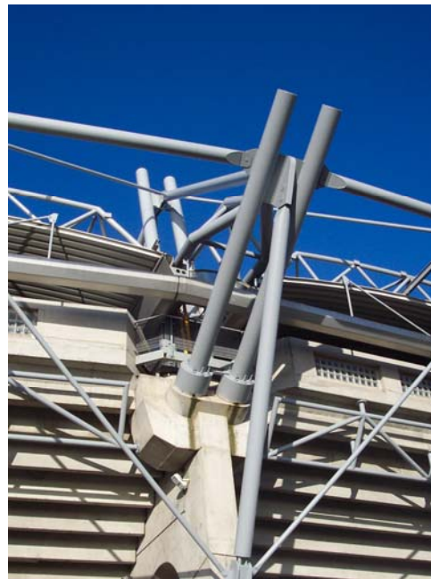
Fig. A-9: The left image shows the cantilever roof structure, the right one the knuckle at the rear of the stadium
