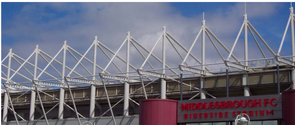
Fig. A-46: West Stand roof from outside
