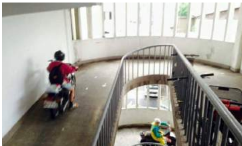
Fig. 10 Spiral parking ramp
