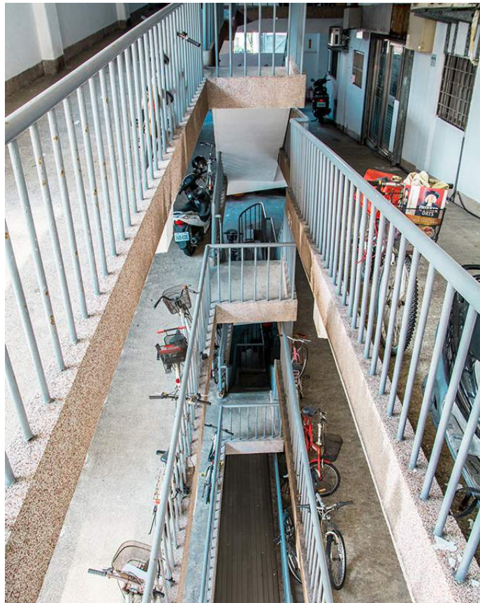
Fig. 11 External access spiral parking ramp with apartment units
