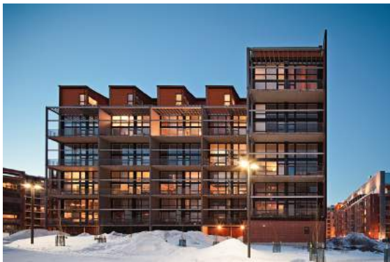
Fig. 20 external appearance of Tila Housing
