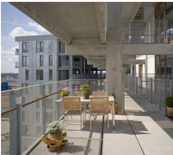
Fig. 7 Externally located corridor access
