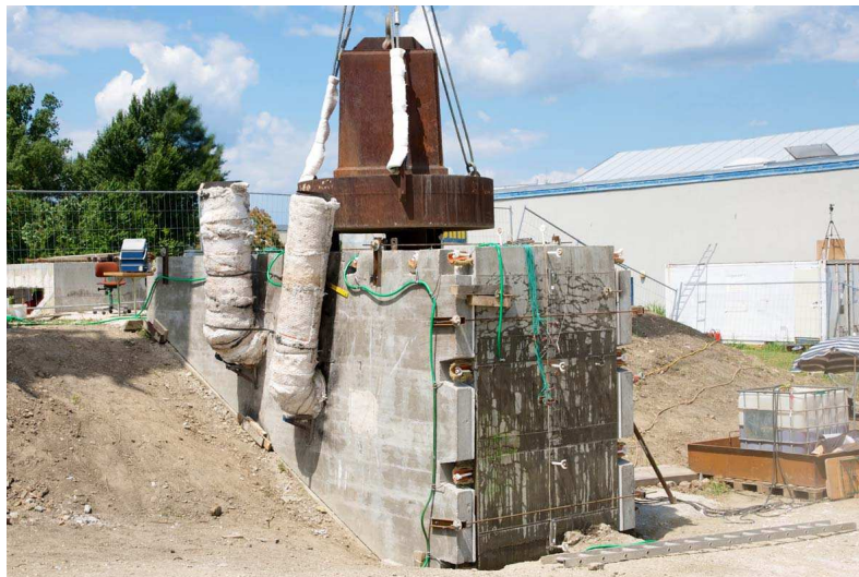
Figure 6: Test setup in large-scale fire experiments (steel weight applied on closed fire chamber)
