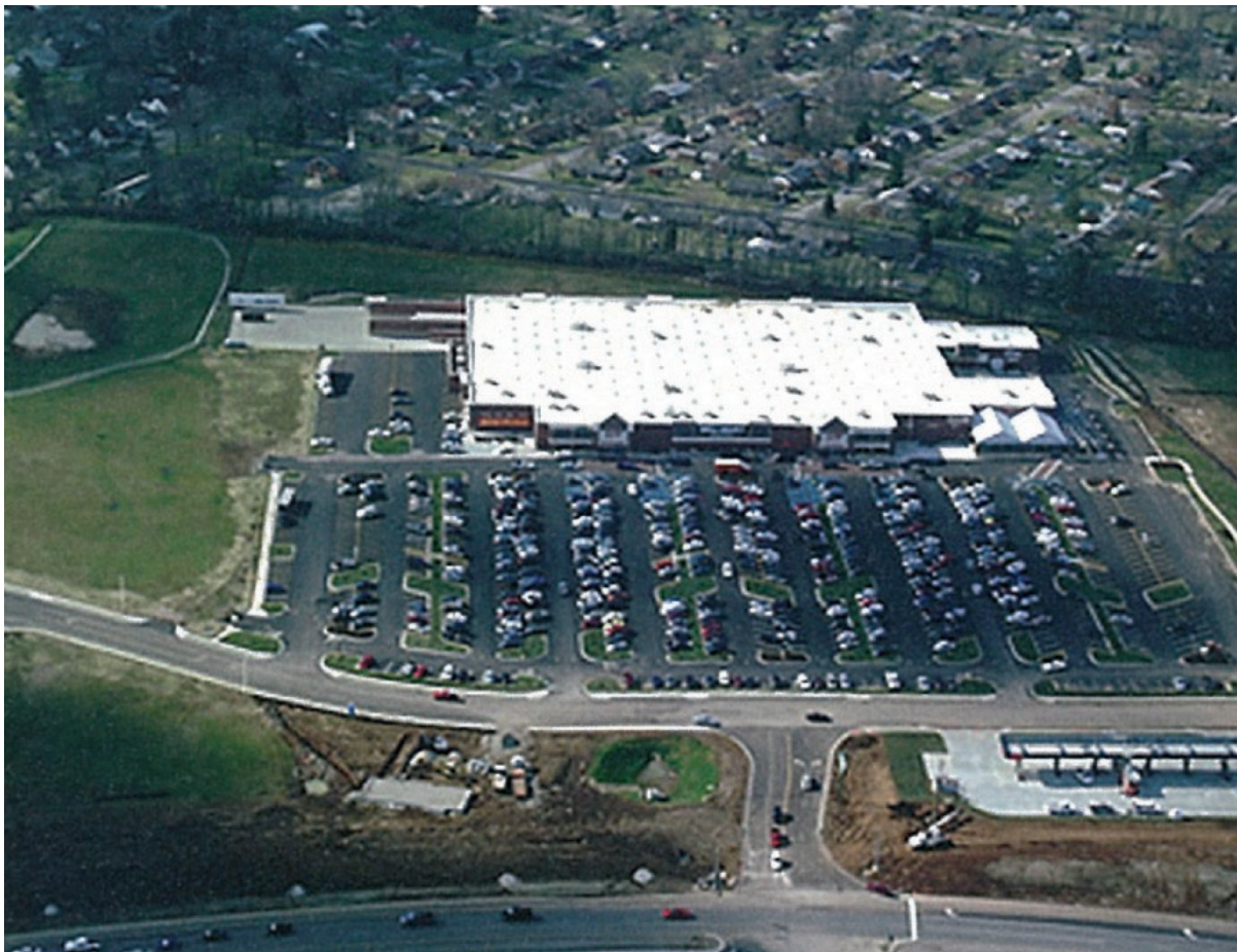
Fig. 3.07 Parking Lot in front of a Walmart, Paris, Kentucky
