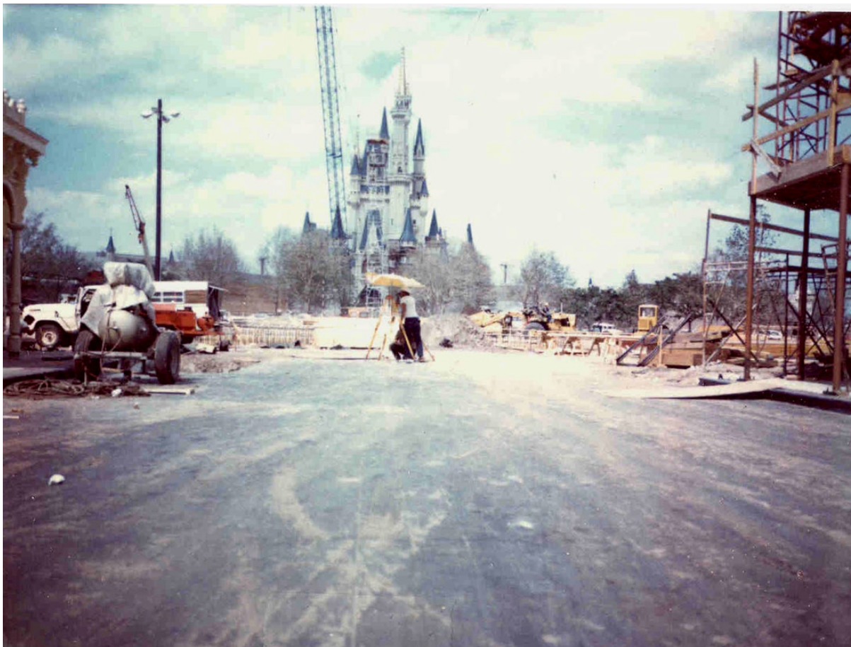
Fig. 3.10 Main Street under construction
