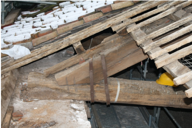
Illustration 62 Truss3 south end
