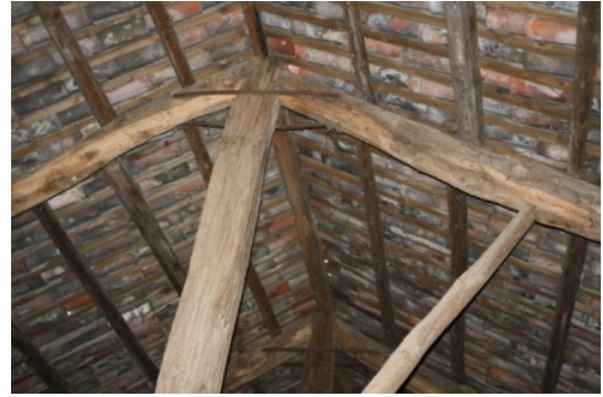
Metal elements connection king post - rafters
