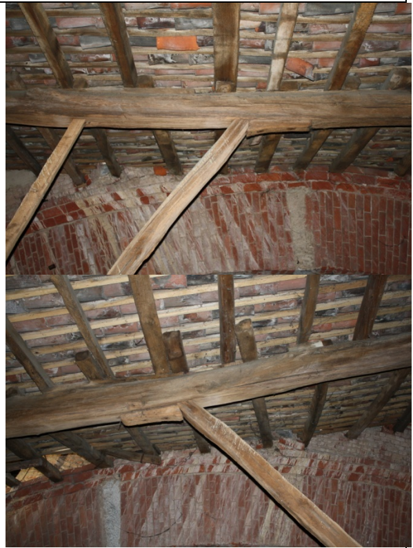
IMG_0739 / IMG_0736 Knot (rafter - chord member)
