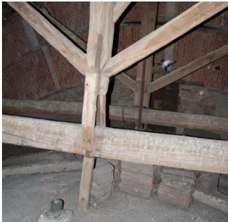
Timber element to avoid displacements
