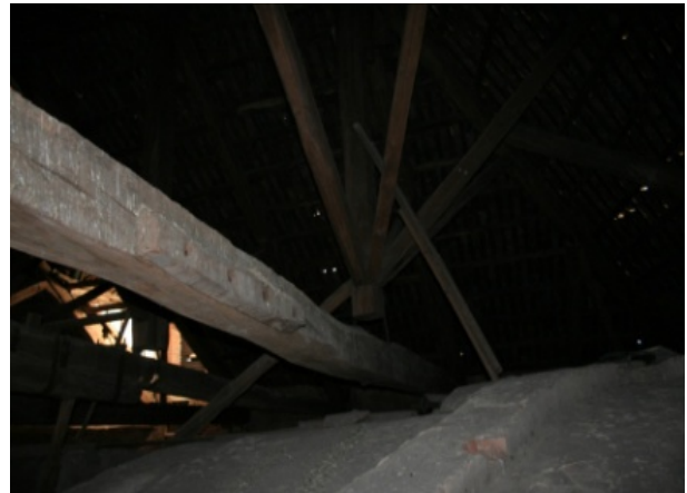
strut to overtake the forces coming from the umbrella structure
