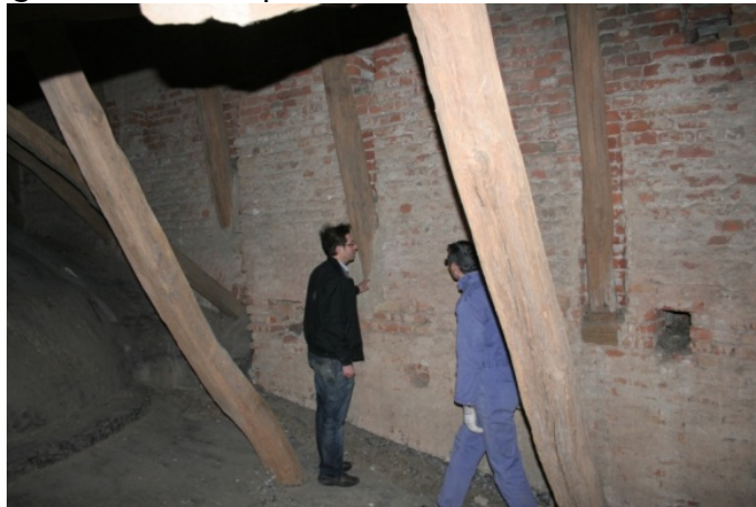
original bearings and bearings which have been closed with concrete
