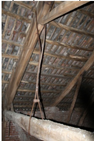
Support tie beam
