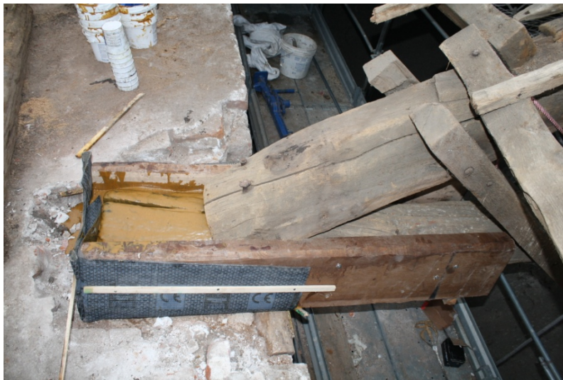
Illustration 60 Truss 2 south end
