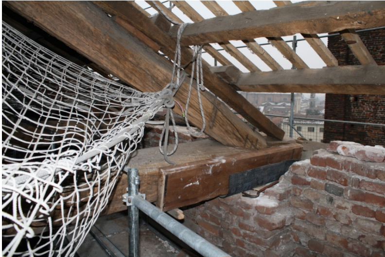
Illustration 61 Truss2 north end
