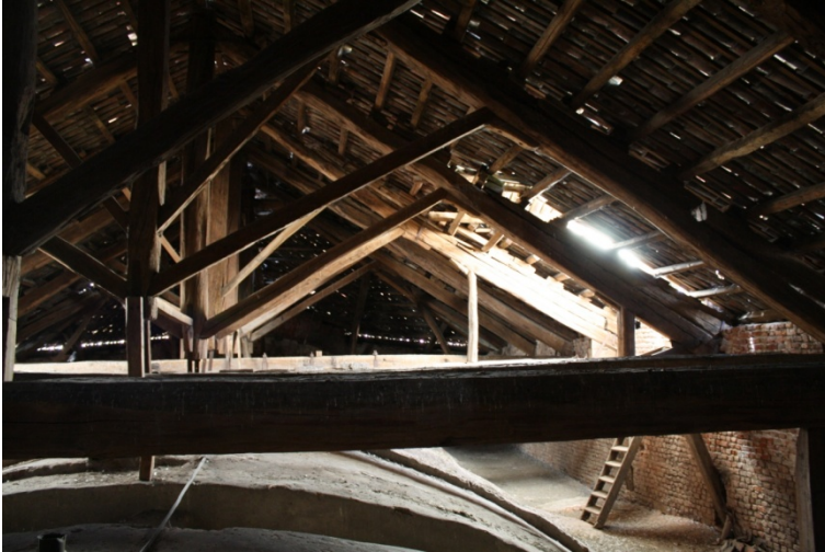
1 main aisle trusses
