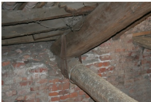
Closed bearing truss
