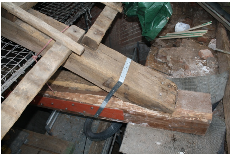
Illustration 58 Truss 1 south end
