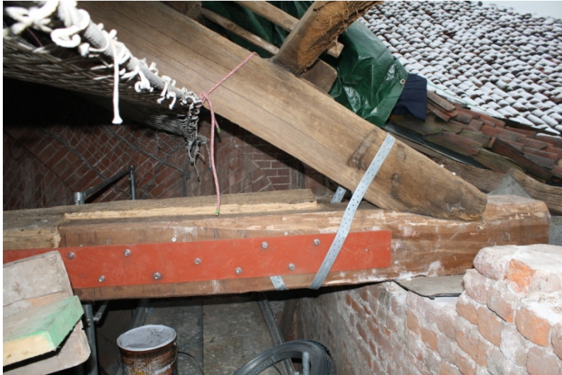
Illustration 59 Truss 1 south end
