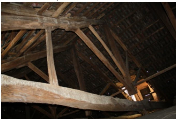
Strut supporting rafter
