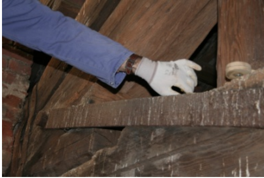
resistance of the surface (screwdriver)
