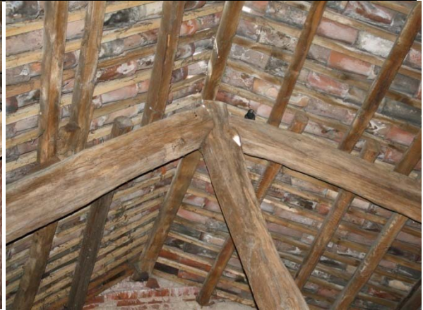
IMG_0735 Knot (king post - rafter)
