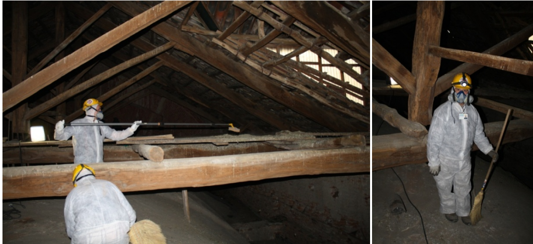
Illustration 52 Company Ecologica cleaning the roof
