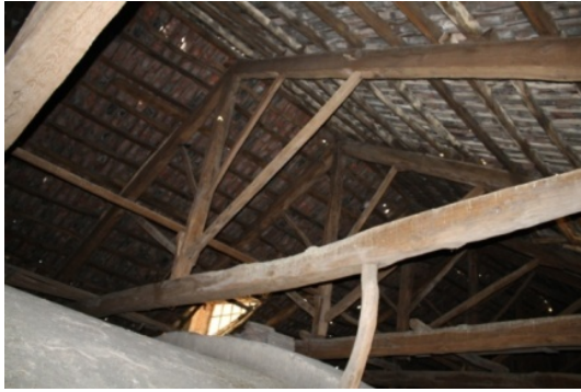
Strut bearing on vault
