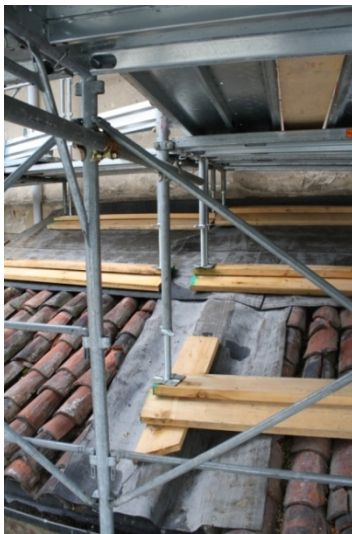
How the scaffold is bearing on the roof
