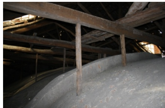
support tie beam (struts bearing on the vault)
