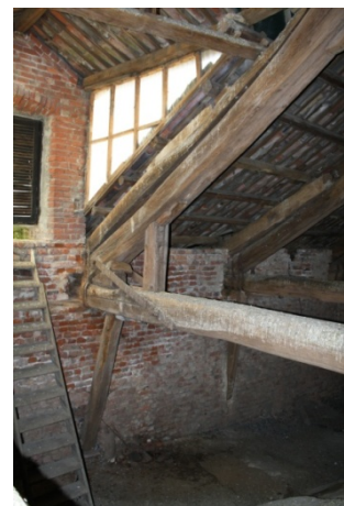
connection rafter - tie beam
