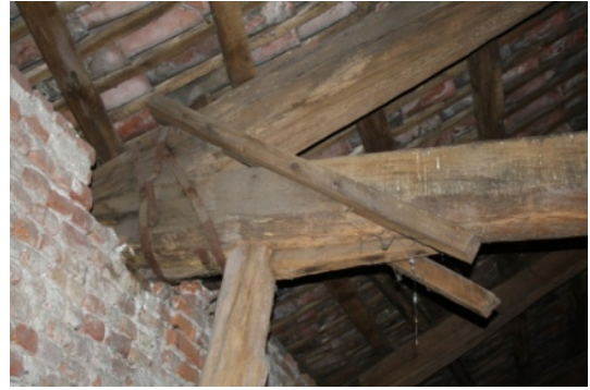
connection rafter tie beam
