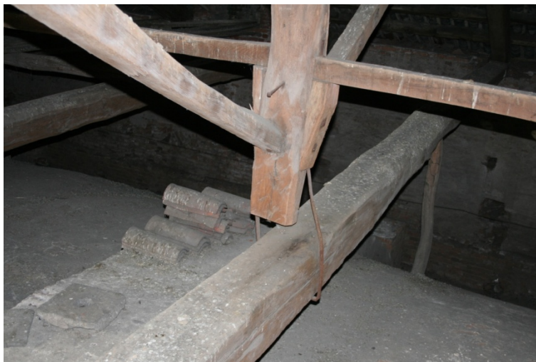
Illustration 69 metal connection
