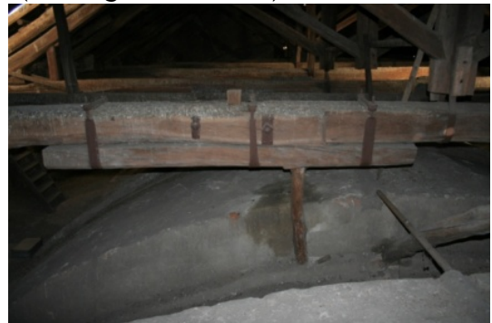
support tie beam
