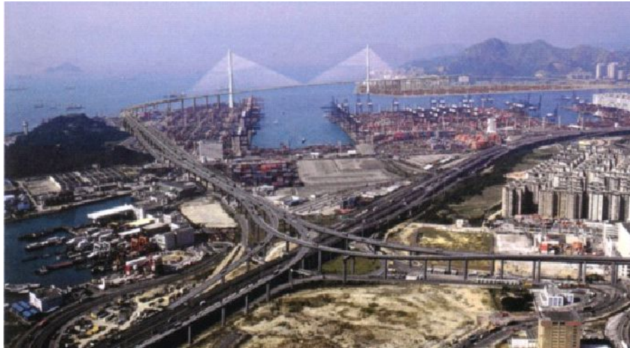
Abbildung 2.4: Stonecutters Bridge (Foto: www.structurae.de )
