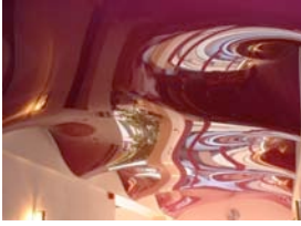
Figure 2.15: Stretch ceilings consist of PVC-foil and allow individual composition in terms of color and surface.
