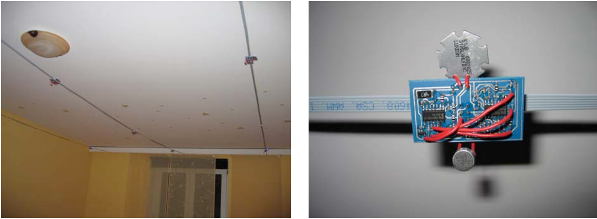
Figure 3.19: Installation of the 12 units within the room.
