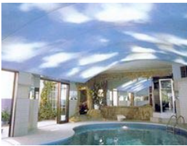
Figure 2.16: A stretch ceiling with paint finish attached to the ceiling above a pool.
