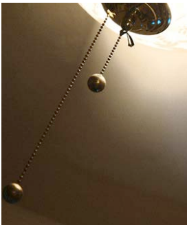
Figure 2.1: Suspended pull cords to control ceiling fan and light.
