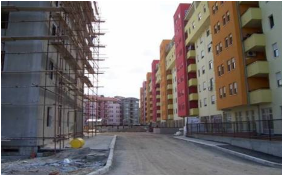
Figure 15 Typical example of 2008 residential construction in Tirana
