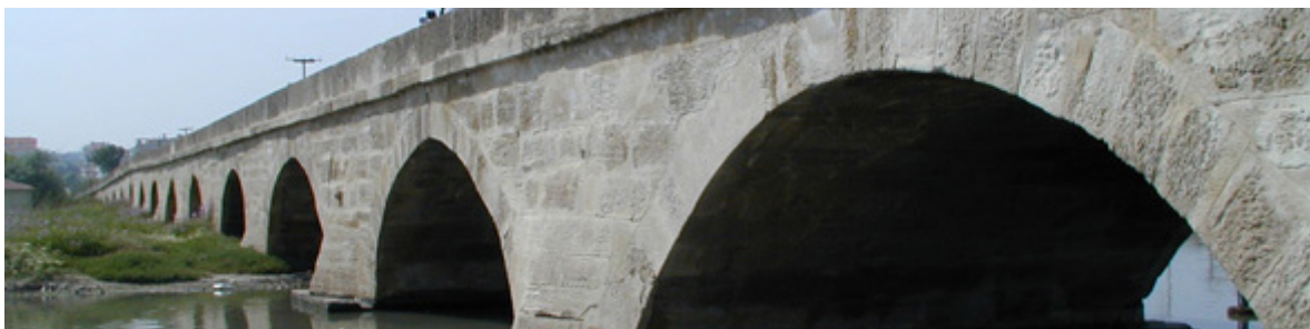
Abb. 19 Süleymaniye-Brücke in Silivri
