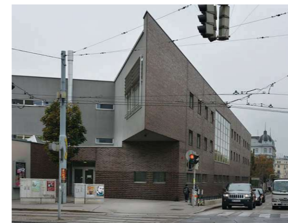
113. Existing condition of the corner (2013)
