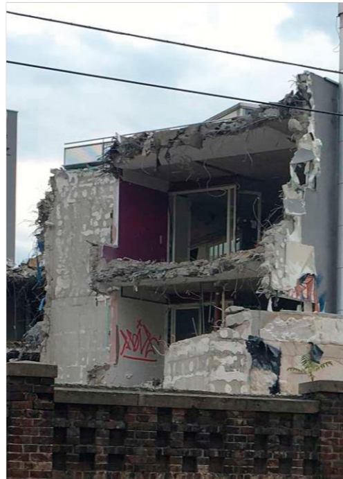
54. Reinforced concrete visible in demolished walls and slabs (2022)
