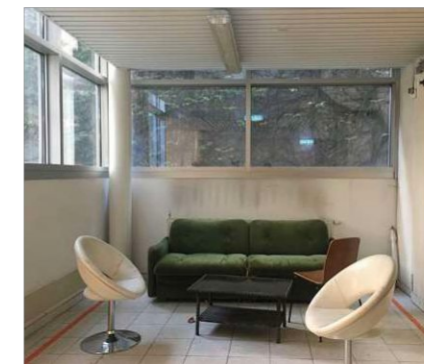
100. Existing condition next to the elevator (2021)
