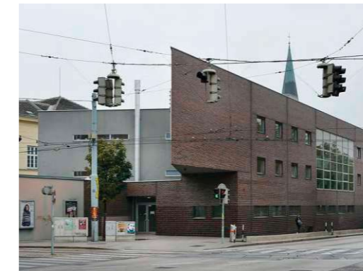
110. The existing condition of the corner (2013)
