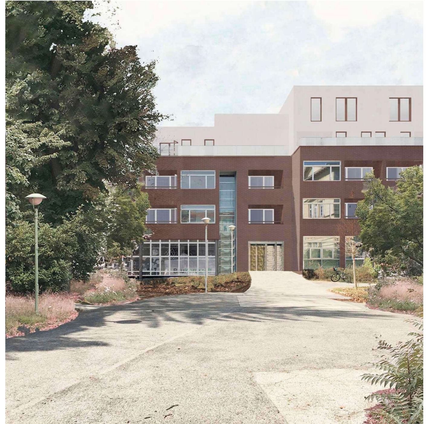
157. The new envelope, the loggias, and the addition
