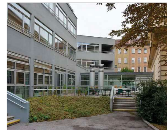
116. The existing condition of the envelope (2013)
