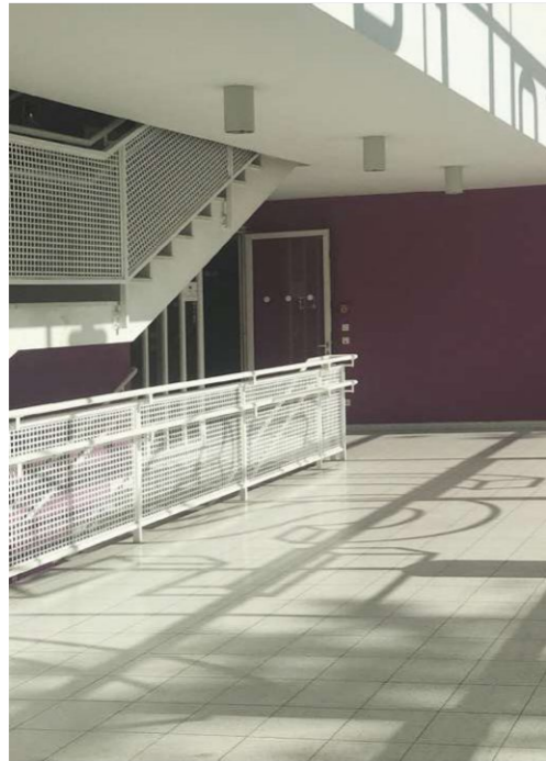
88. White-coated railing with perforated panels on main stairs (2021)
