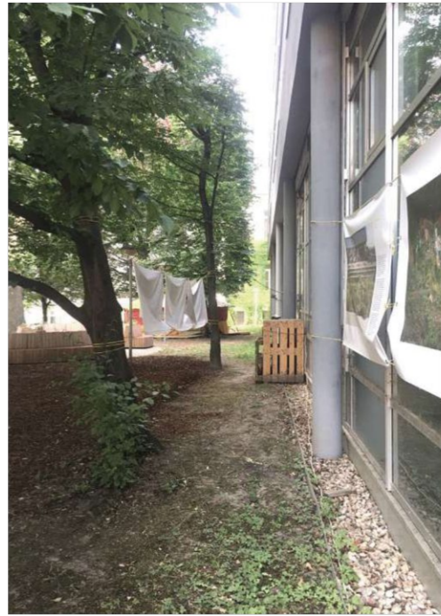
52. Load-bearing columns in the exterior (2021)
