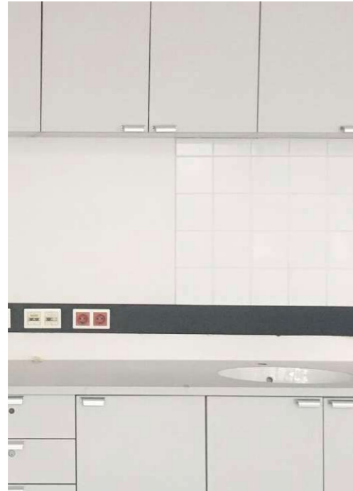
68. White square tiles on plasterboard wall (2021)
