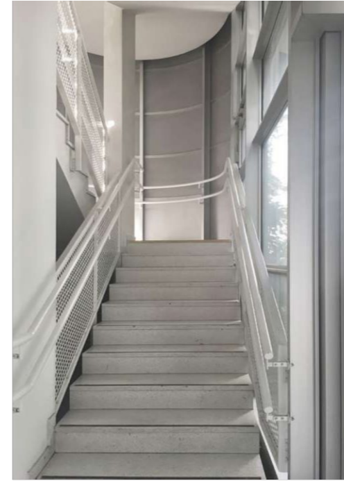
55. Prefabricated concrete two-flight stairs (2021)
