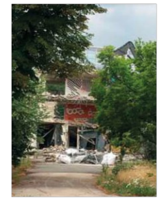
43. View of the demolished Europa-Pavillon from the courtyard (2022)
