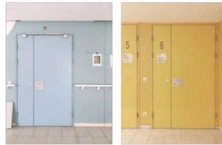
39. Doors into former patient rooms (2021)
