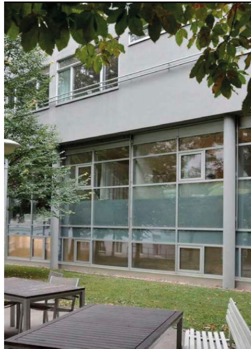
62. East Facade - View from the courtyard (2013)
