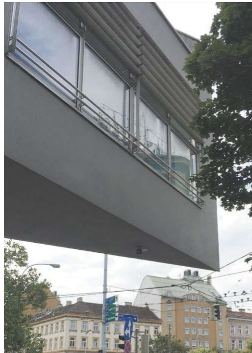
86. Large windows with exterior jalousies in the corner (2021)
