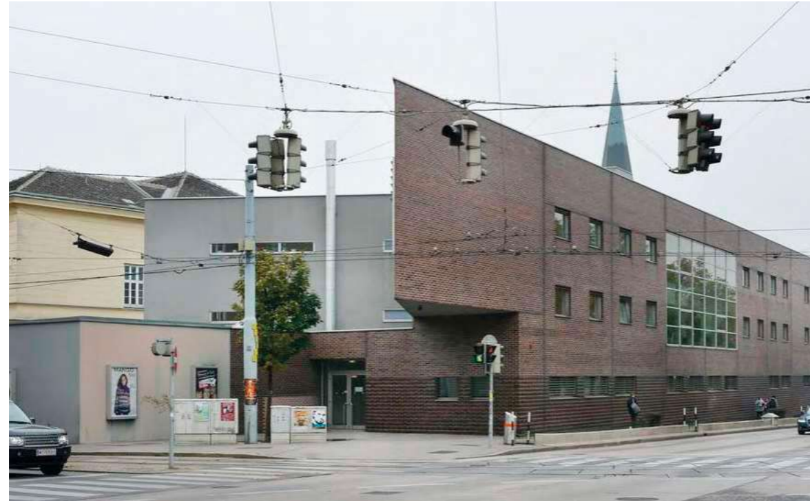
18. View of the north end corner and main entrance (2013)
