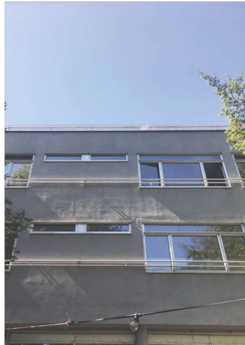
85. Windows with low and high parapets on the courtyard side (2021)
