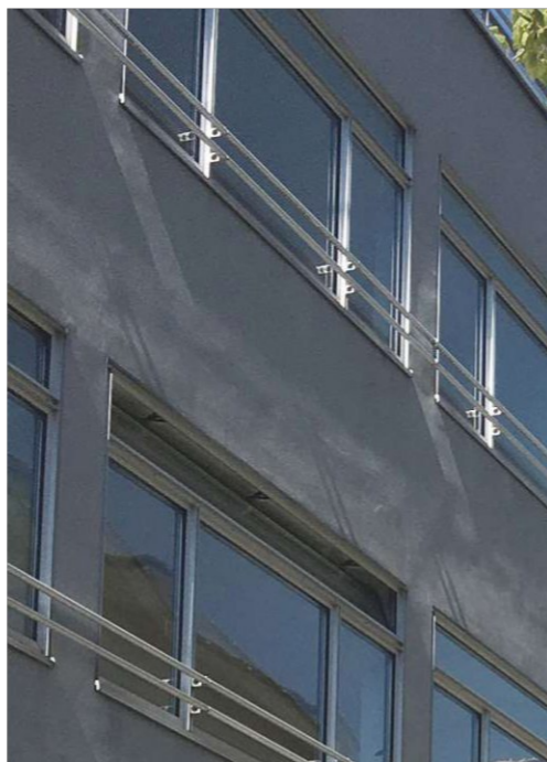
91. Railing as an element of the facade in front of windows with low parapet height (2021)
