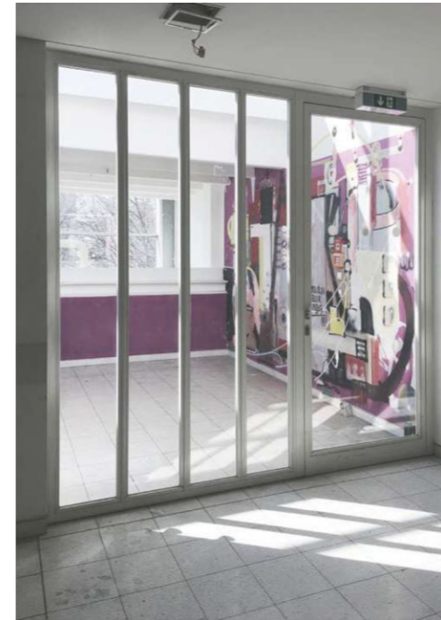
80. Glass and aluminum interior door to stairs (2021)
