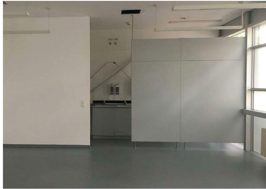
59. Partition plasterboard wall (2021)
