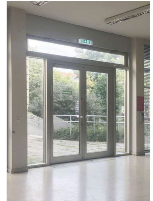
81. Glass and aluminum double-leaf entry door (2021)
