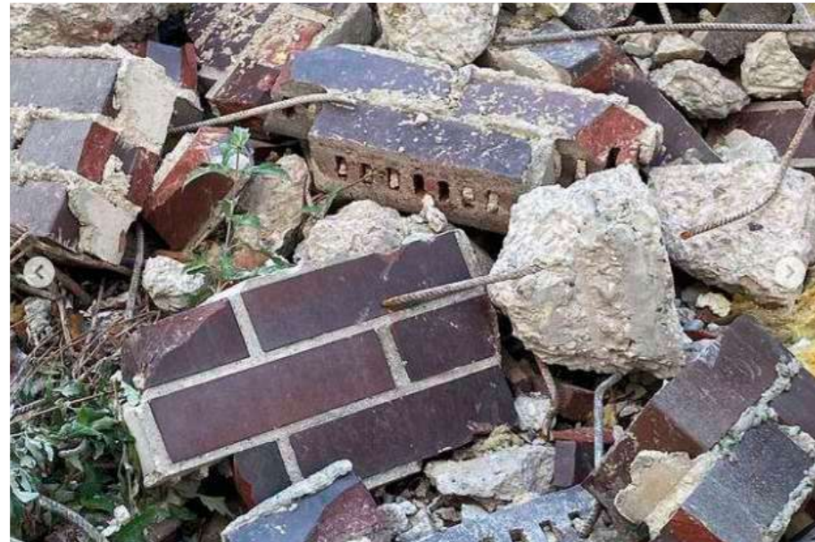
67. The demolished clinker facade (2022)
