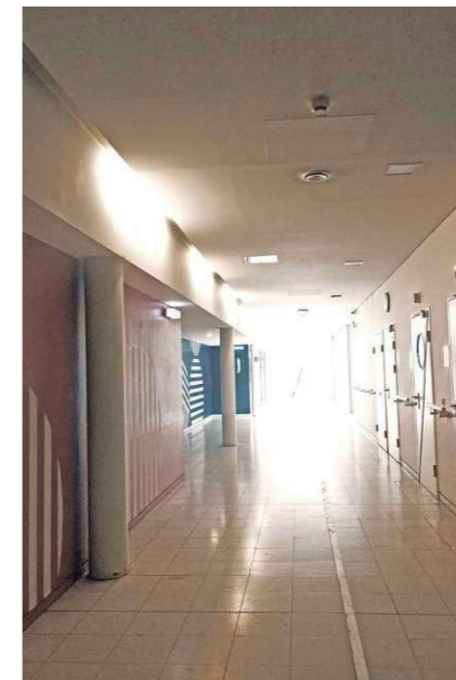
97. Existing condition of the corridor (2021)
