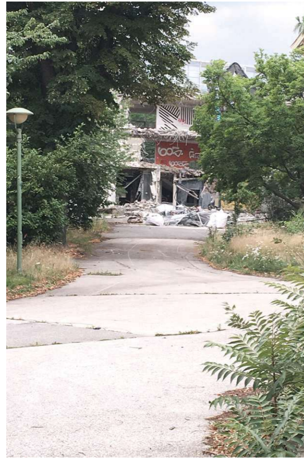
37. View of the demolished Europa-Pavillon from the courtyard (2022)
