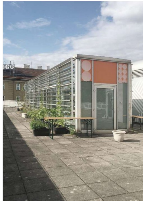
65. Stair to the roof terrace (2021)
