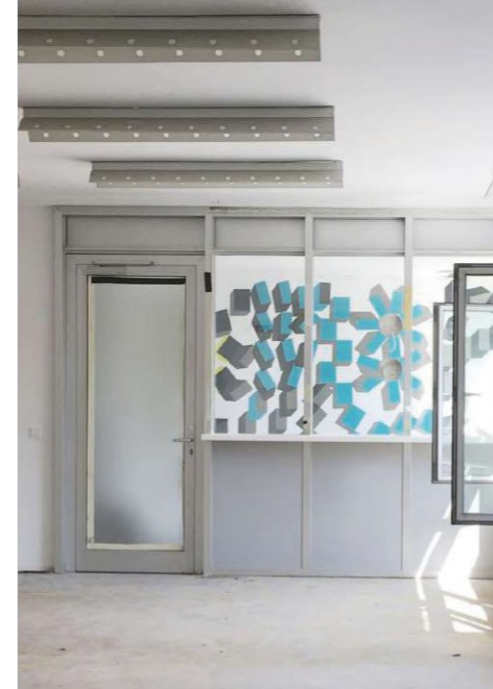
82. Glass and aluminum door to the loggia (2022)
