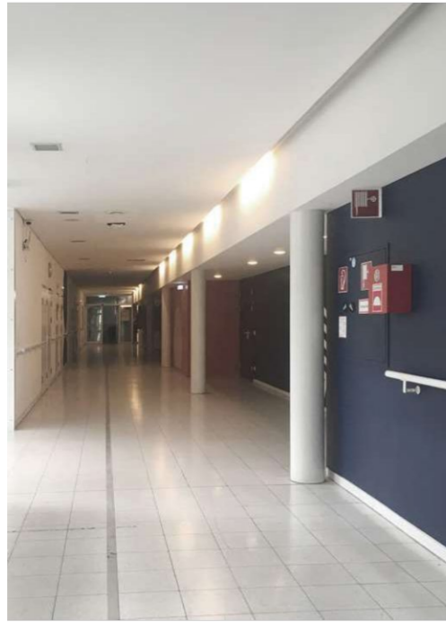
51. Load-bearing columns in the circulation (2021)
