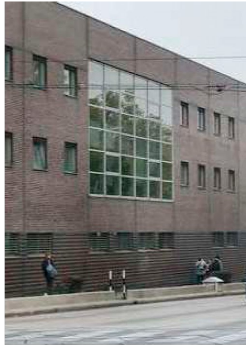
63. West Facade - View from the Neubaugürtel (2013)
