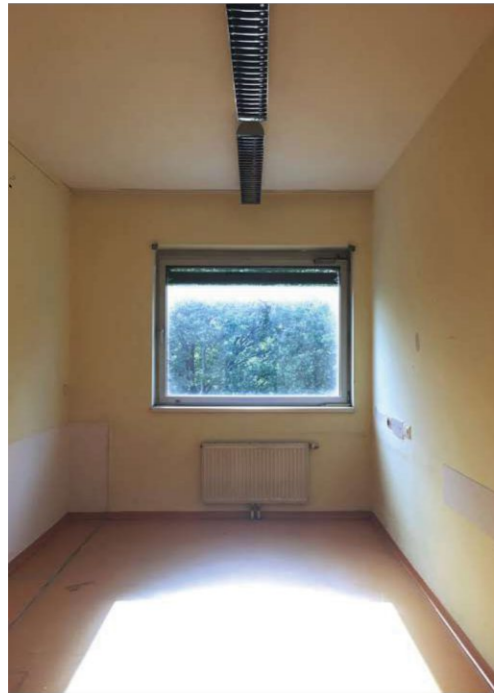
84. Soundproof window with a high parapet on the street side (2021)
