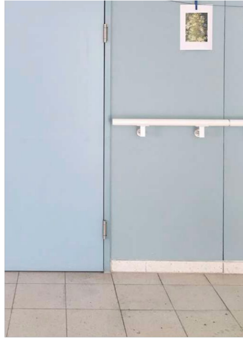
89. White-coated handrail in the corridor (2021)
