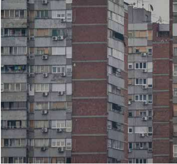
Facade of dense built residential buildings
