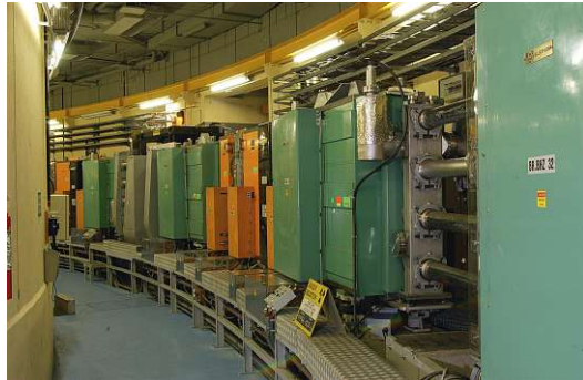
(a) The four PSB rings, with the main dipoles (green) and quadrupoles (orange) [92].
