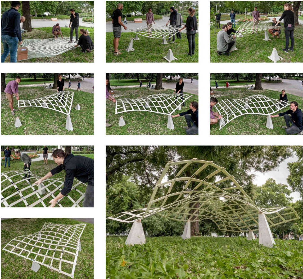
Fig. 3.20: Several steps of the deployment of the EGG model and the deployed structure. The deployment process does not require a lot of force, and the curvature of the structure emerges naturally.
