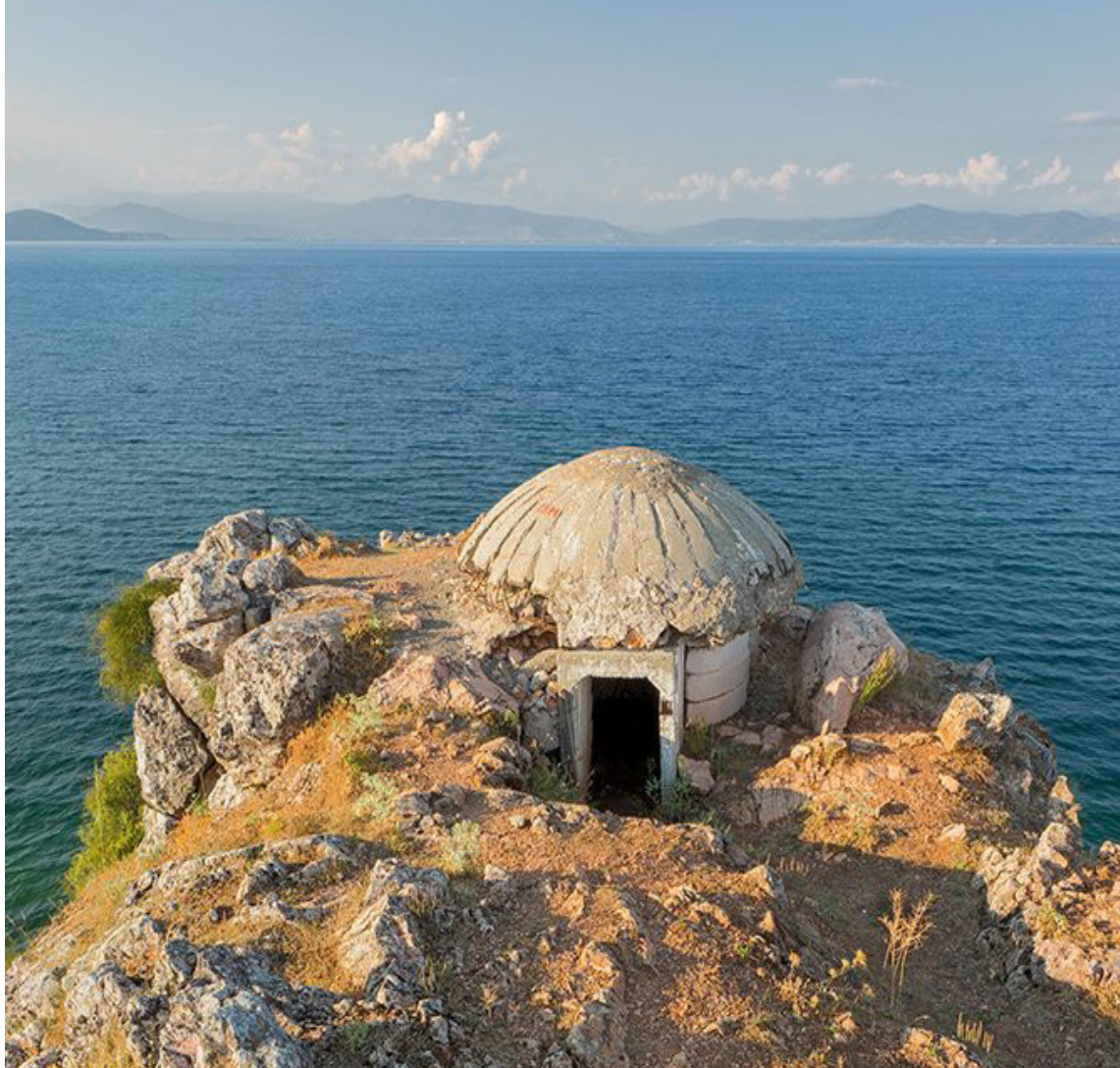
FIGURE 04 BUNKER IN THE EDGE OF LAKE OHRID, 1975-1990
