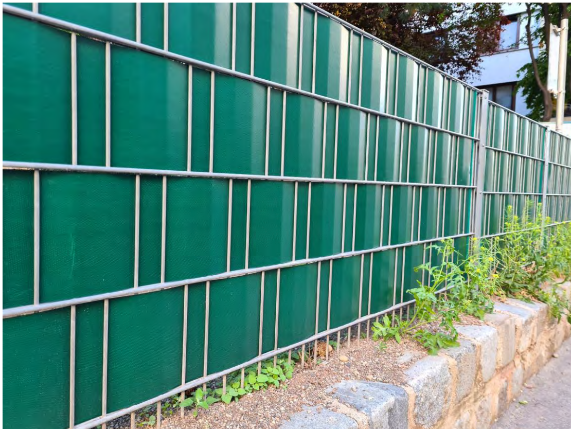
Figure 17. Typical privacy screen foil applied into a typical double wire mesh fence at the dog zone of Rudolf-Sallinger-Park in the fifth district of Vienna. (own photo, taken on May 18 th 2022)
