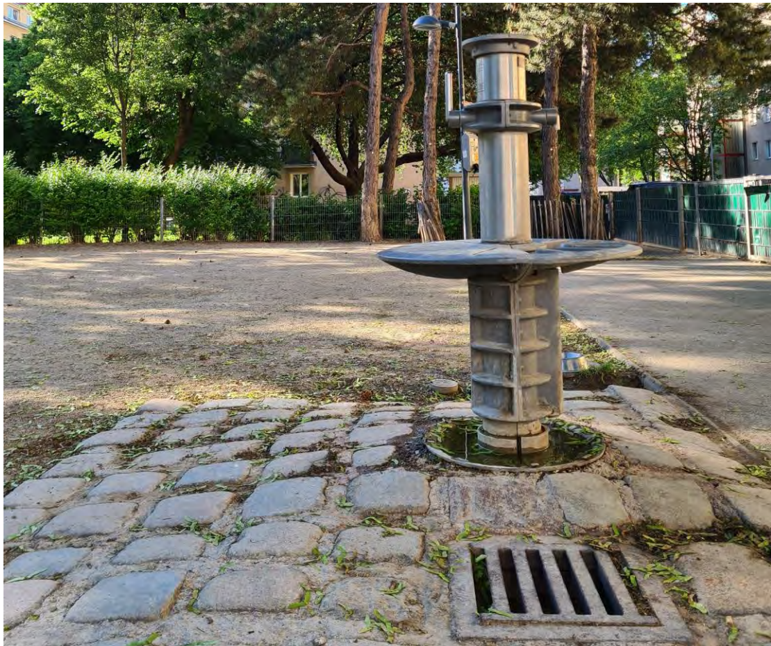
Figure 31. Drinking fountain in the dog zone in Leopold-Rister-Park in the fifth district of Vienna. The area around a drinking fountain is designed so that water does not stay lying. (own photo, taken on May 18 th 2022)
