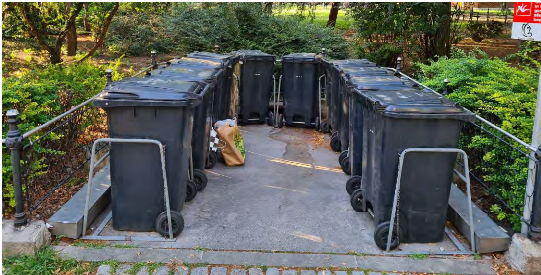
Figure 2. The former “dog toilet” at Brigittaplatz (cf. Eckl & Ramharter 2006: 86) is now used for keeping rubbish bins. The infrastructure of the former dog toilet can be seen to this day: water was sprayed from the metallic elements on the sides of the former dog toilet and the dog waste was flushed into the gutter which can be seen between the two rubbish bins in the back. (own photo, taken on June 19 th 2022)
