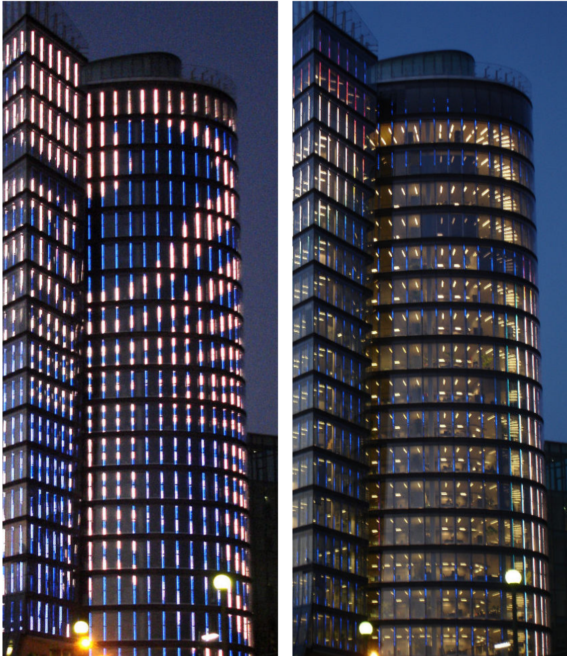
Figure 2.1: Room lighting interfering with media façade projections. In the left picture the effects shown by the media façade are clearly visible. In the right picture the effects are barely visible because the room lighting of the building is interfering heavily.
