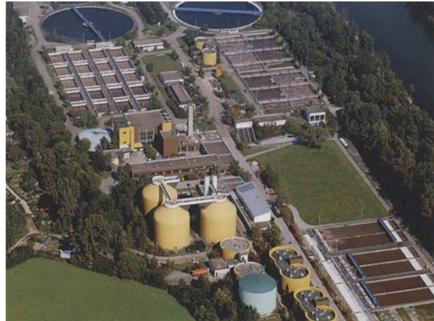
Figure 5-4: Aerial view of wastewater treatment plant in Augsburg (Stadt Augsburg, 2006)
