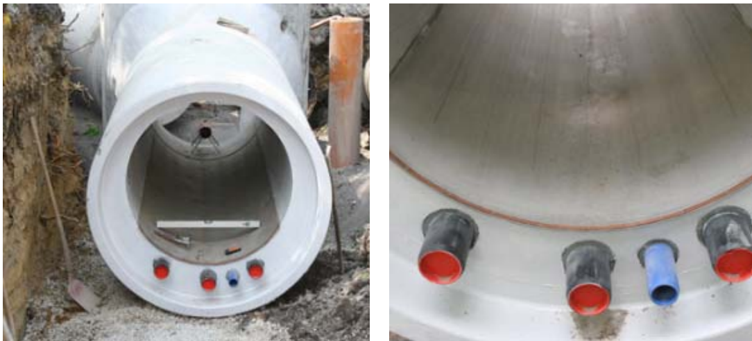
Figure 3-5: Integrated RABTHERM heat exchanger modules (Wallstein, 2009)
