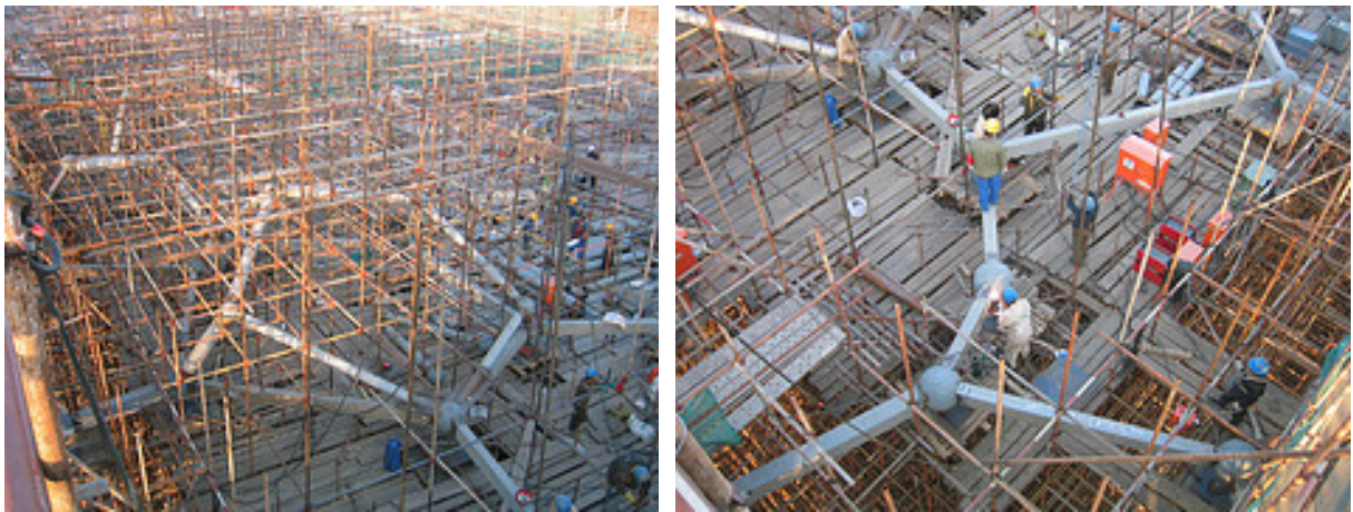
Figure 28: Picture of roof nodes during the assembly of the structure
