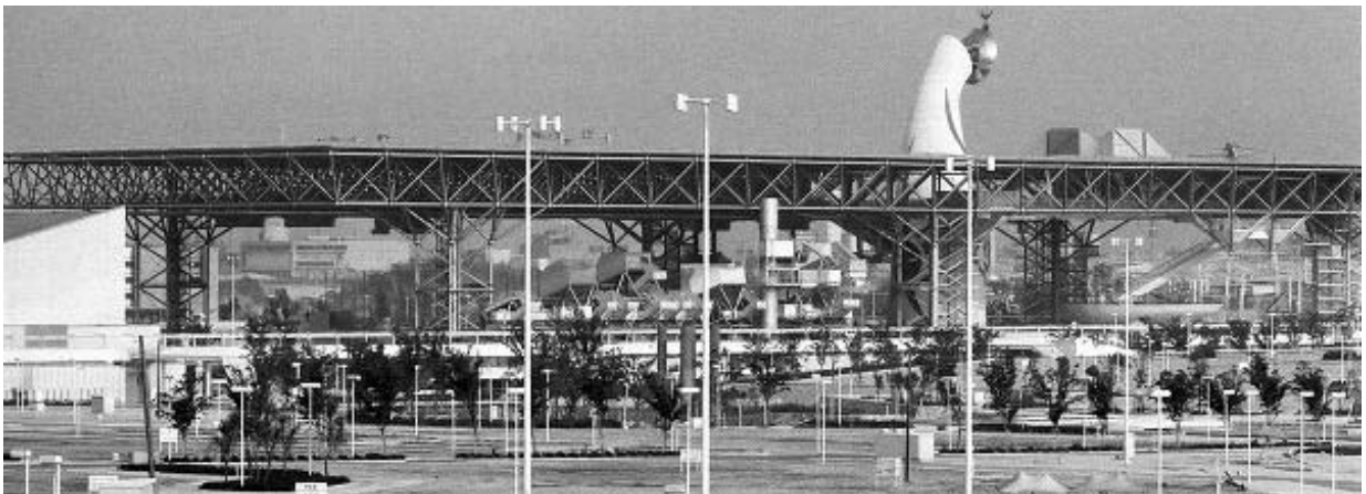
Figure 36: The roof structure of the Symbol Zone supported on six columns
