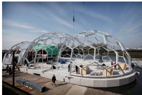
Figure 6.2: Floating pavilion, Rijnhaven, Rotterdam[7]
