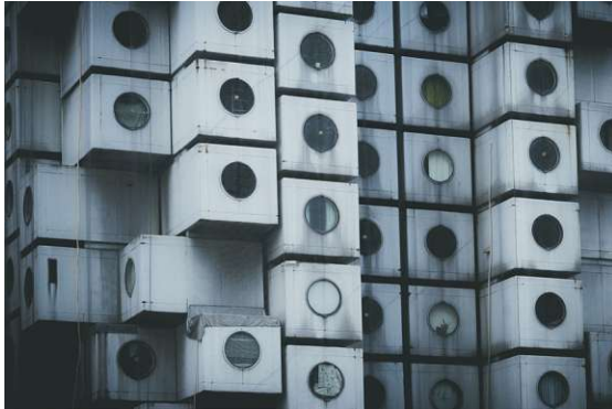
Figure 9.5: Kisho Kurokawa Architect and associates Nakagin Capsule Tower. 1972
