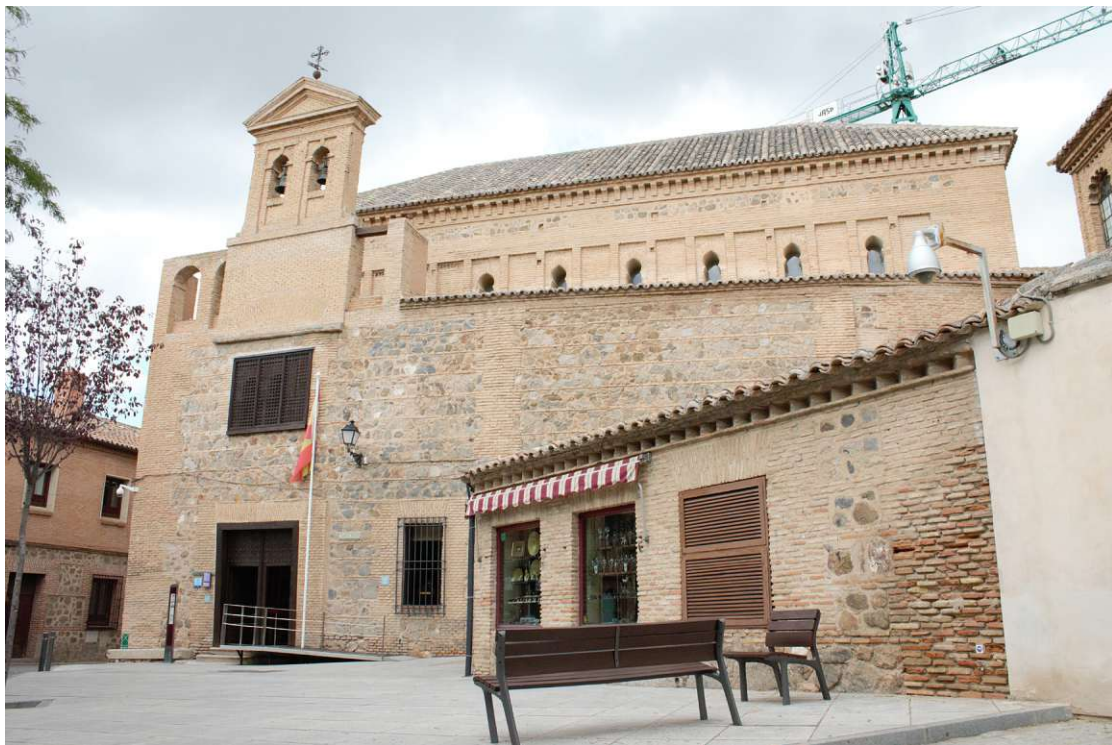
Fig. 15 Southern Façade, Synagogue of the Transit
