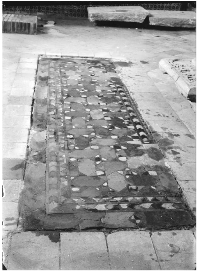
Fig. 125 Photo of the discovered tile flooring that belongs to the medieval synagogue's tevah, Moreno, n.d.
