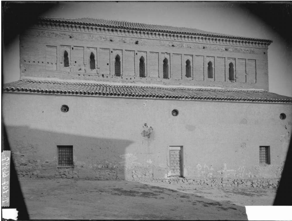
Fig. 36 View towards the Northern Volume – Vernacci, n.d. : The exterior wall of the annex building in north was stayed with cables and the partition walls were formed following the vault to unify the three exhibition rooms after the restauration work in the beginning of nineties
