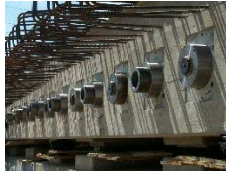
Abb. 96 Festanker (SUSPA DSI GmbH, 2008)
