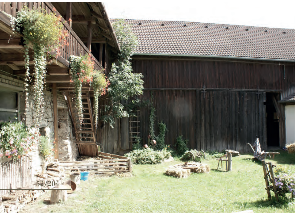
Abb. 35: Hofraum am Prannleithen-Hof in Yspertal
